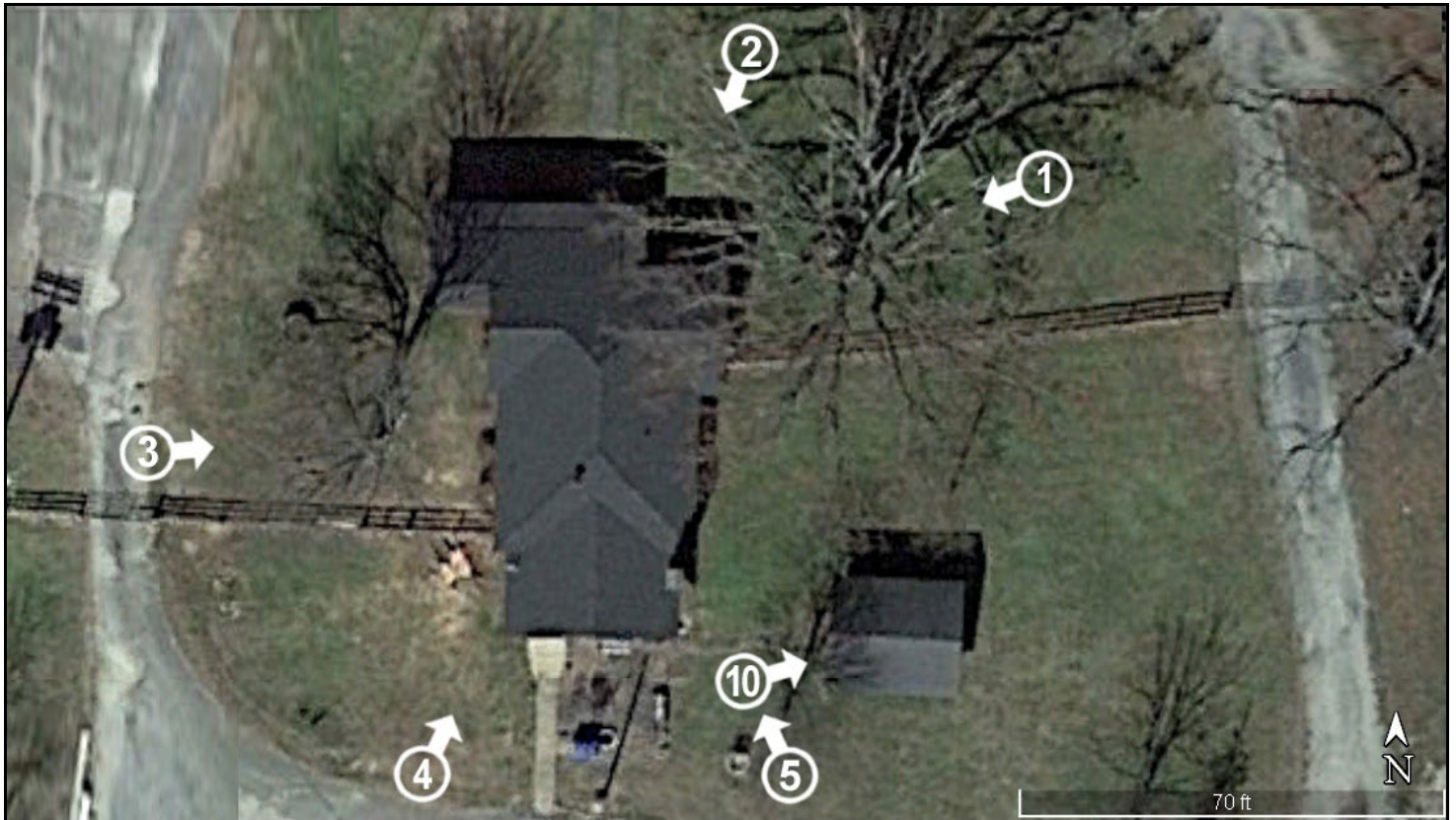
Haywood County Farm Superintendent's Residence Aerial Photolog
