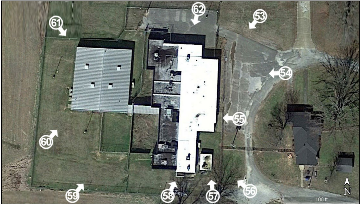
Haywood County Jail Aerial Photolog Exterior
