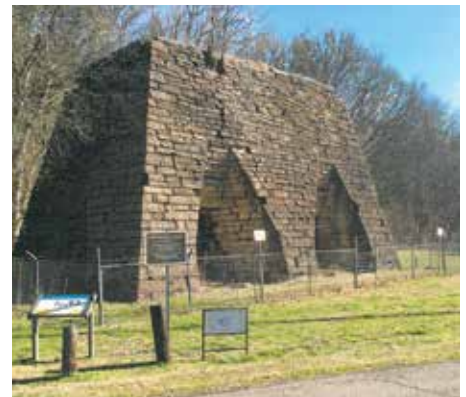
Perry County in Perry County, for using a Historic Preservation Fund grant to clear invasive trees, vines, and lichen that threatened the structural integrity of the limestone battered walls that comprise the Historic Cedar Grove Furnace and Spring House.
