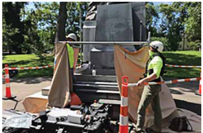
Vandalism in 2020 required the removal of spray-painted graffiti from the base of the monument
