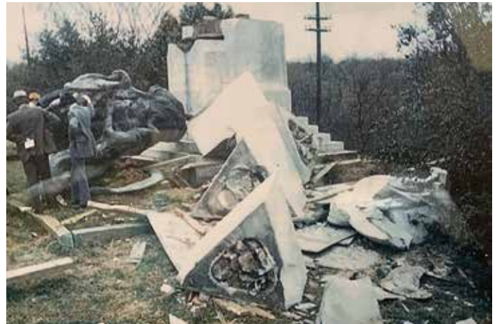
Tornado damage in 1974 required full restoration of the bronze sculpture and recreation of the destroyed obelisk
