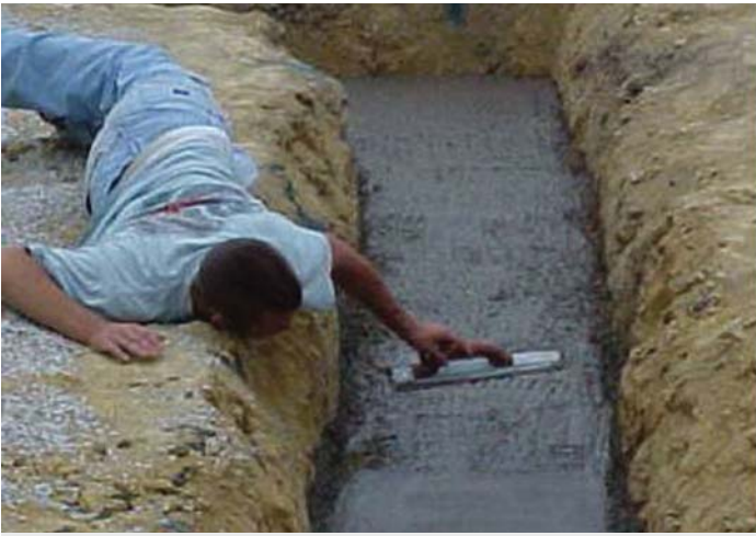
B. The concrete on top of the footer is leveled to establish a surface for the foundation of the home. Once the footer has hardened, the perforated drainage pipe will be laid on the outside of the poured foundation wall. The reinforcing rods were positioned in the trench before pouring the concrete.
