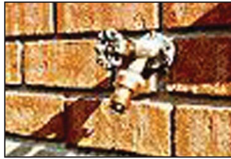
Figure 9.17. Hose Bib With Vacuum Breaker
