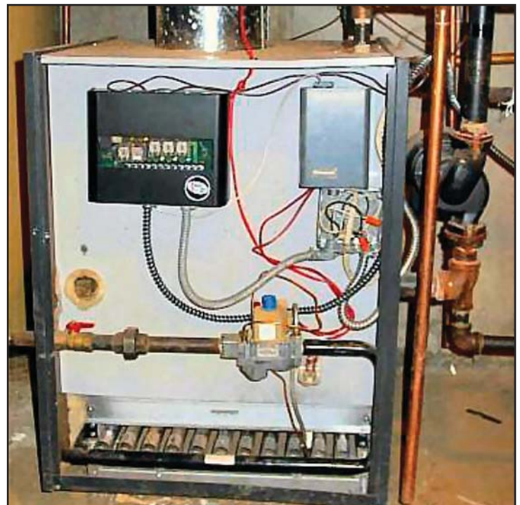
Figure 12.9. Gas-fired Boiler
