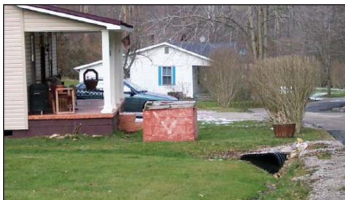
Figure 8.7. Typical Dug Well
