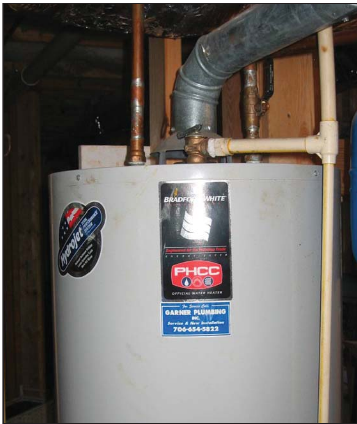
Figure 9.4. Temperature-Pressure Valve
