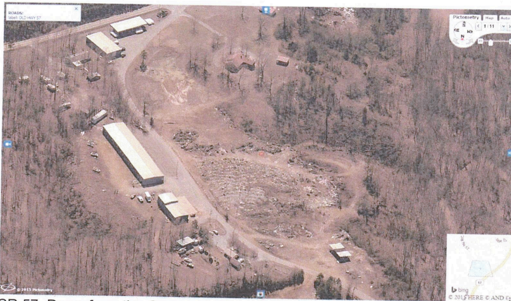
SR 57, Down from the Corner of 57 South on SR 57, GPS: 35.029184 -88.236498 Or 35°1'45.0624" N – 88° 14' 11.3928" W
