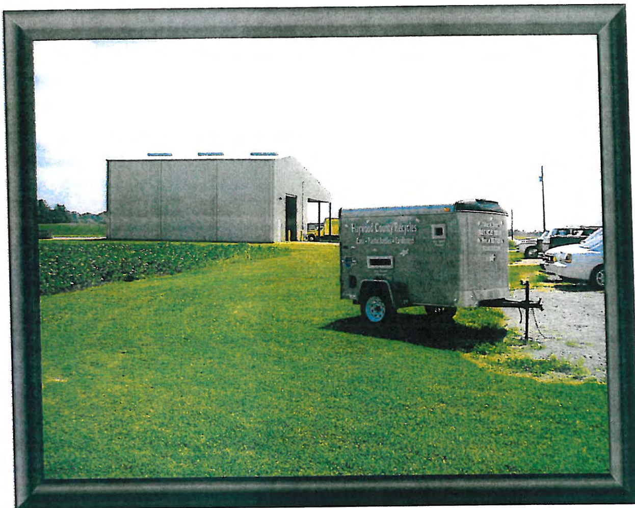
The Haywood County solid waste complex is well-designed with plenty of room for expansion. The Haywood County Landfill is the only Class III/IV operating in Haywood County but has more than 100 years of use expectancy remaining.
