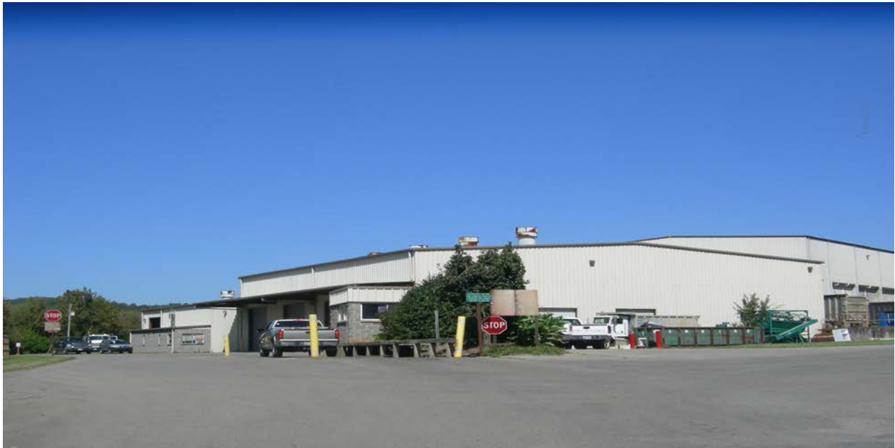
Greenville/Greene County Transfer Station
