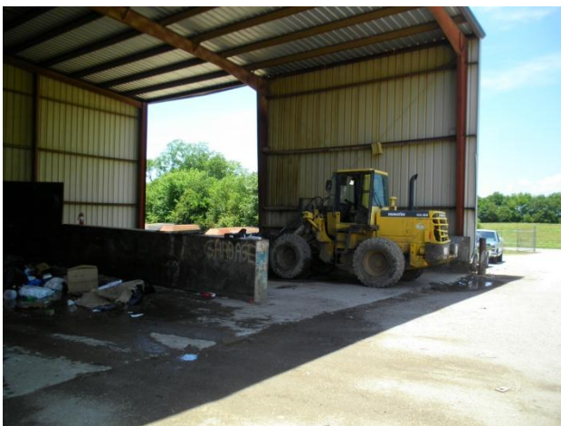
Franklin County Solid Waste Transfer Station 487 Joyce Lane, Winchester, TN
