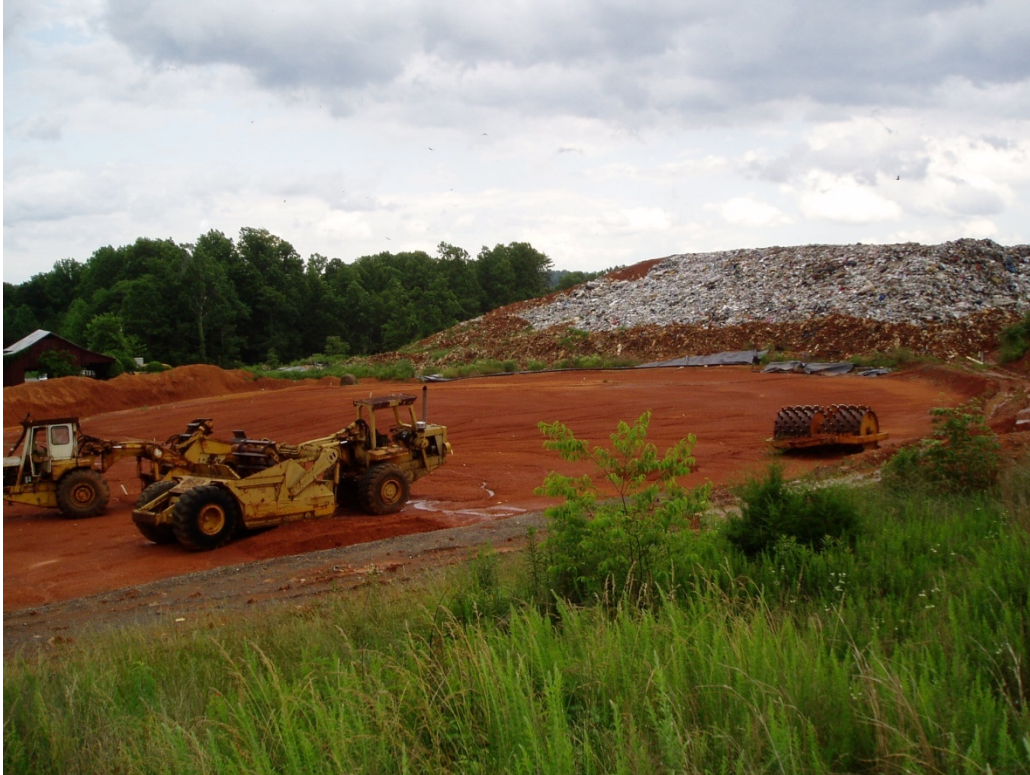
Working on New Cell at Upper Cumberland Landfill
