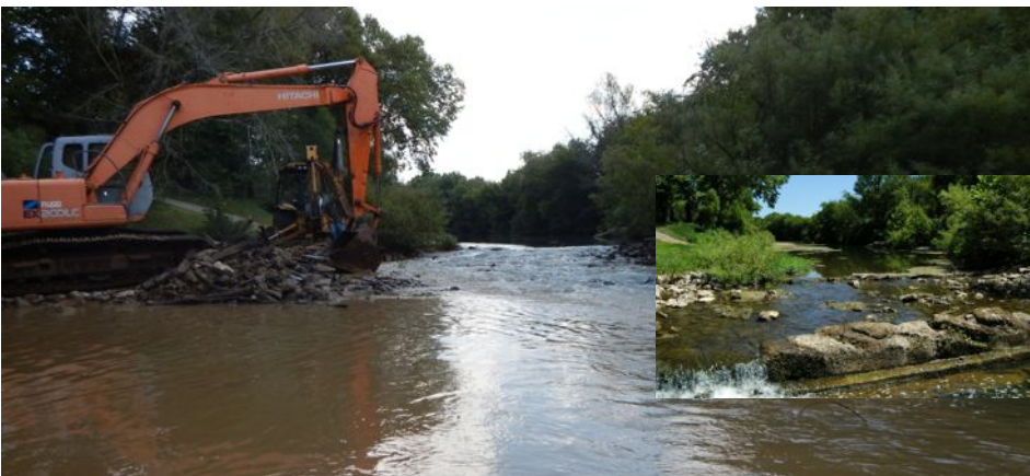
Removing Brown's Mill Dam, inset: dam before removal - Pandy English, TWRA
