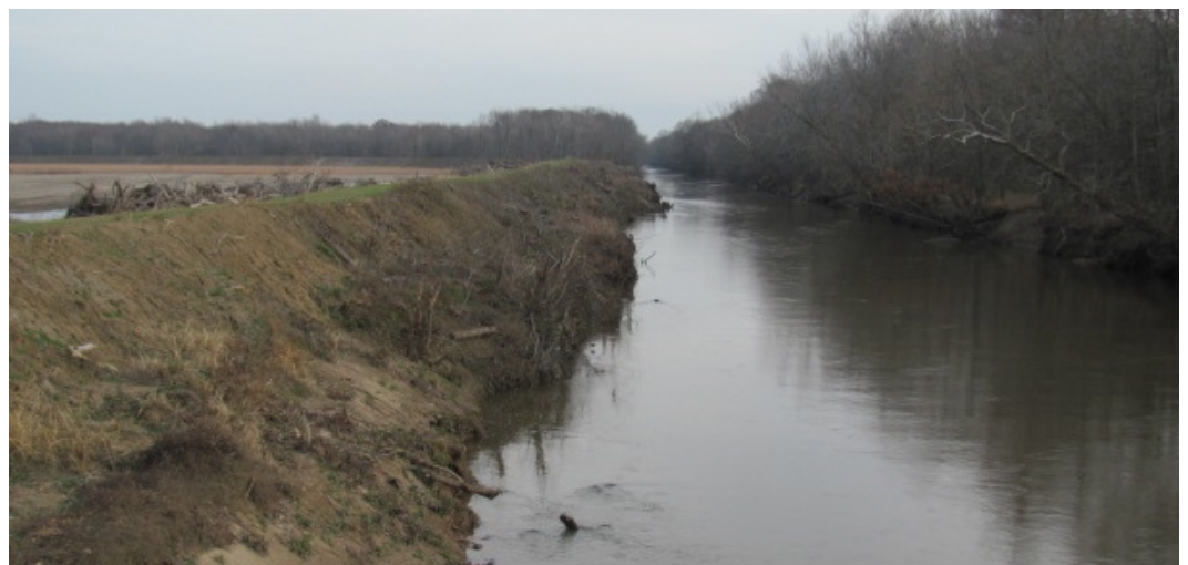
A channelized stream in west Tennessee, South Fork of the Forked Deer River - Rob Colvin, TWRA
