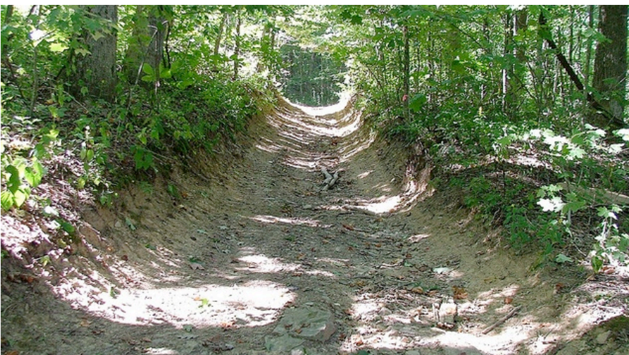
Logging road in Tennessee: best management practices help to mitigate erosion, concentrated flows, and sedimentation. - Chris M. Morris
