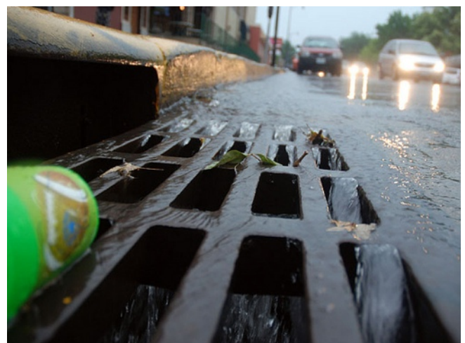
Urban Drains carry pollutants; impervious road surfaces increase runoff and destabilize normal stream flow. - KOMU News
