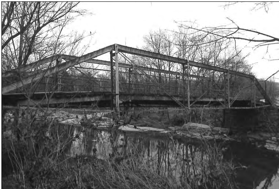
Figure VII-06: The Buena Vista Ford Bridge spanning Lick Creek Smith County (#56, 80- A0206-00.47) is an atypical Pratt truss with fishbellied bottom chord built in 1907 by the W.T. Young Bridge Company (above). In 1986 TDOT removed the truss span (top next page) and lifted it off its original abutments and moved it on a truck to Loudon County (middle next page). This view shows it on a tandem truck negotiating a curve in rural Smith County. The City of Loudon renovated the bridge for pedestrian use on a city trail (bottom next page).
