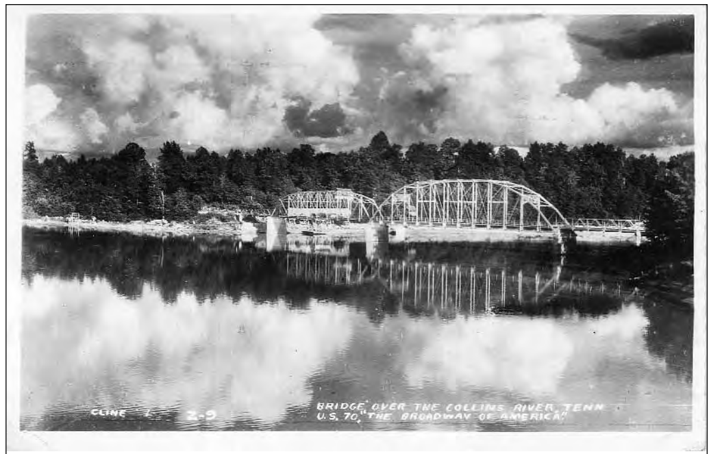
Collins River Bridge: Also once scheduled for demolition, the Collins River Bridge (#112, 89-04261-11.60) at Rock Island in Warren County is now part of a trail system in the Rock Island State Park (Author's Collection).
