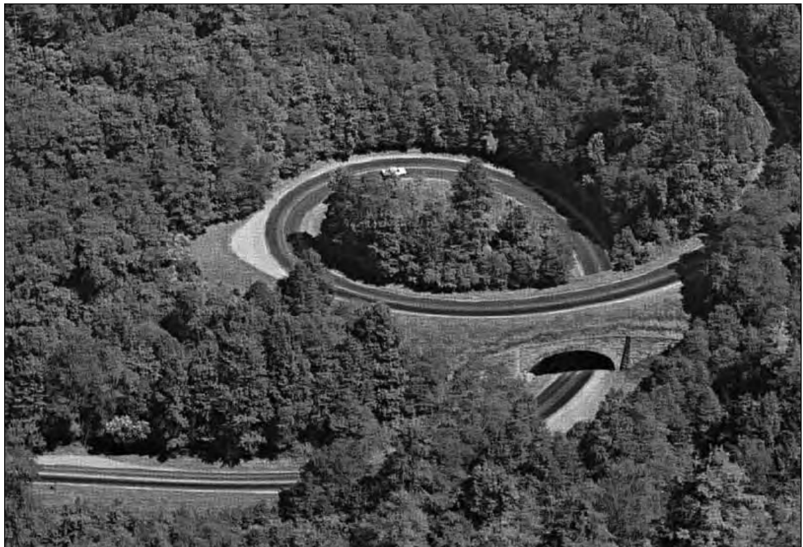
Aerial View of the Loop (sometimes called a "corkscrew" or "pig-tail" bridge).
