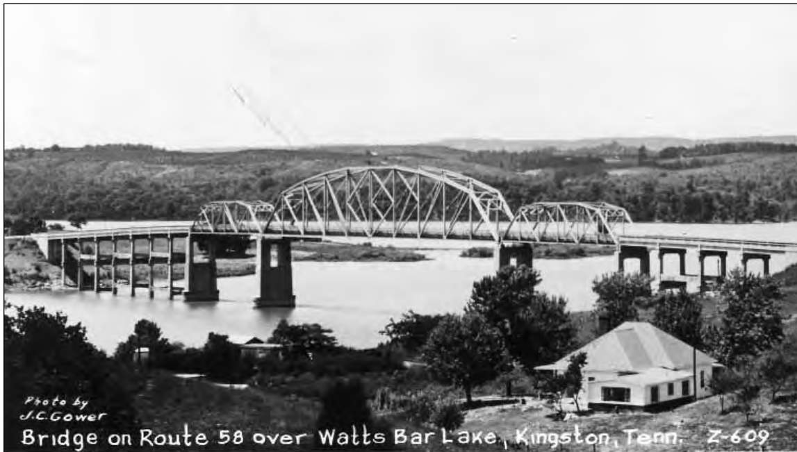
Figure II-49: Postcard view of the Calvin J. Ward Bridge on SR58 spanning the Tennessee River near Kingston, (#130, 73-SR058-11.92). Note the toll house in the lower right corner (Author's Collection).
