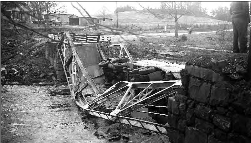
Figure II-70: Collapse of unidentified bridge with truck in Tennessee (TDOT Photo Collection).
