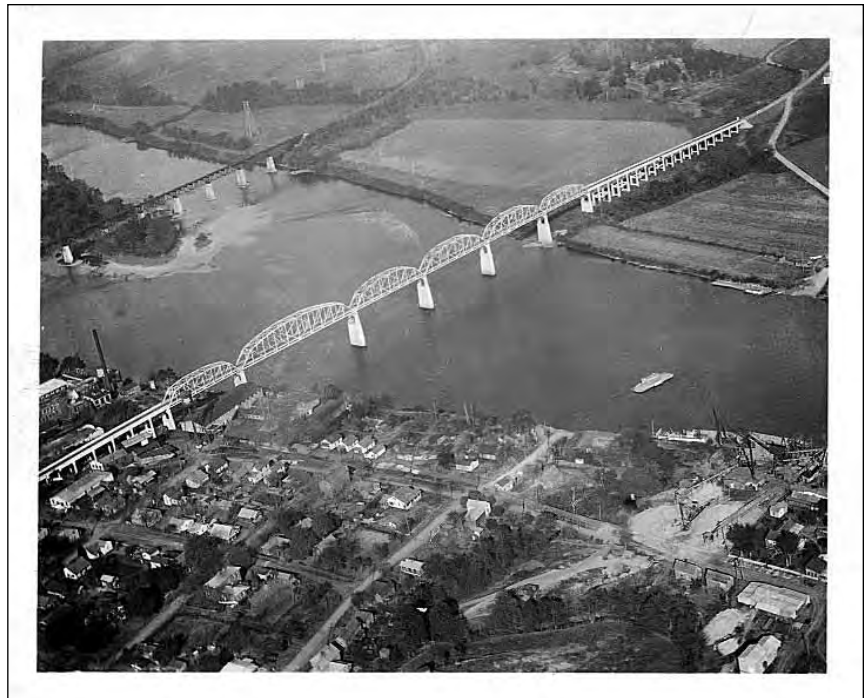
Figure II-50: 1930 aerial view of the Loudon Bridge spanning the Tennessee River. Note the ferry on the right side of the photo. In several instances, the ferries charged a lower rate than the state run bridges, and some ferries remained in operation until the toll bridges were freed (TDOT Photo Collection).
