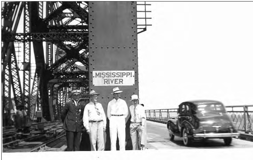
Figure II-31: Circa 1940 photo of the Harahan Bridge with cantilevered vehicular lanes (#77, 79-NonHighway-4) (TDOT Photo Collection).
