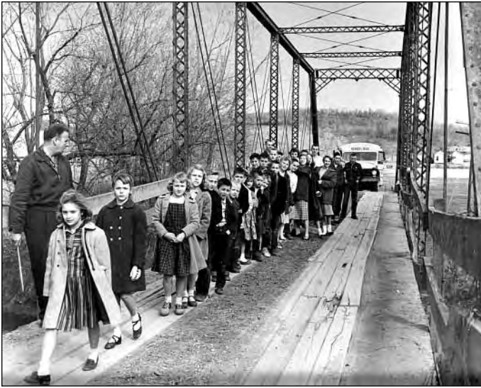
Figure II-69: Photograph showing children exiting a bus to walk across a dilapidated bridge near Pulaski in Giles County. The bus driver then drove the bridge across the bridge and the children got back on the bus. Scenes like this occurred across the country twice a day as counties faced increasingly dangerous older bridges (Courtesy, Tennessee State Library and Archives).
