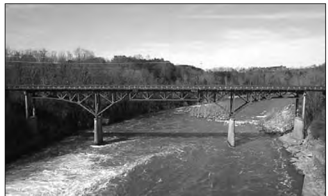
Figure II-54: Elevation view of the Oscar Lovette Bridge in Greene County (#138, 30-SR070-08.48).
