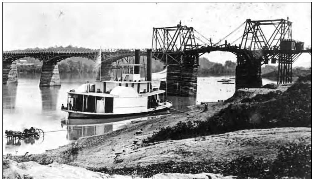
Figure II-06: Military Bridge from the Civil War era spanning the Tennessee River at Chattanooga, Hamilton County (Courtesy, Chattanooga Hamilton County Bicentennial Library Collection).
