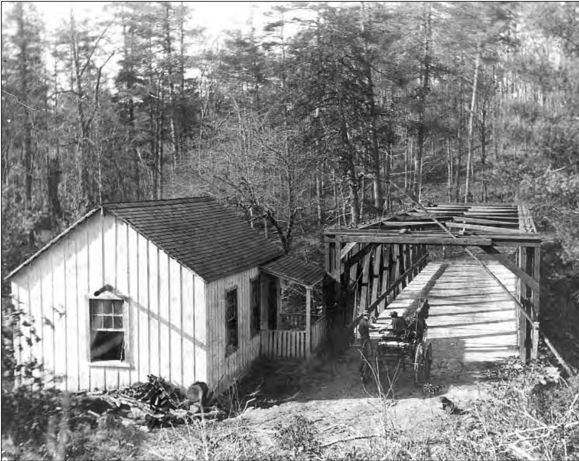
Figure II-05: Toll house and wood and iron through truss bridge at Rugby, built circa 1880; (Courtesy, Tennessee State Library and Archives, MG149, B18,F5). Today, the abutments from this bridge hold a 1920s truss bridge, (#7, 65 NonHighway 1) which TDOT has bypassed and left in a small pull-off.
