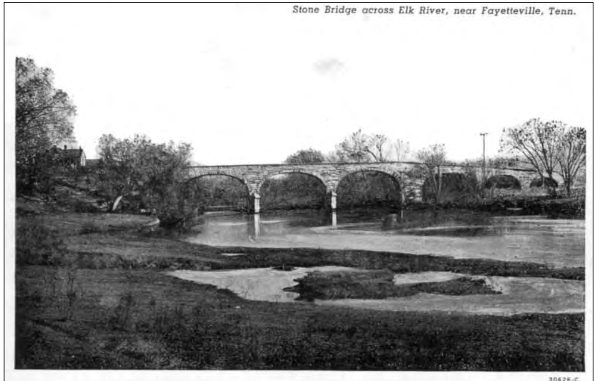
Figure II-08: Old Stone Arch Bridge over the Elk River, Fayetteville, Lincoln County (Author's Collection).
