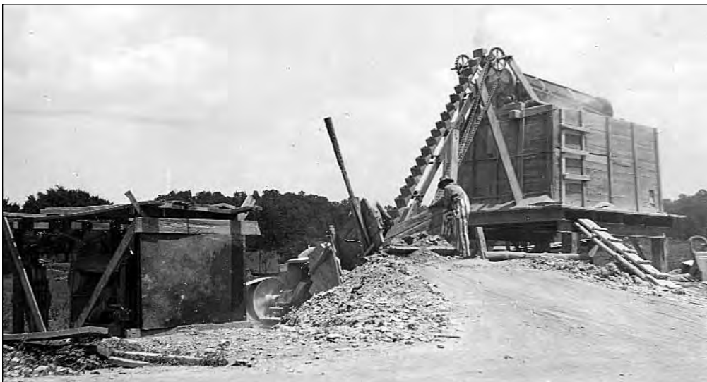
Figure II-10: Undated photo of prisoners working the “crusher” on a road project in Meigs County (TDOT Photo Collection).
