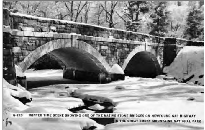
Elevation view of the Walker Camp Prong Bridge (#144, 78-SR071-05.23) in the winter.
