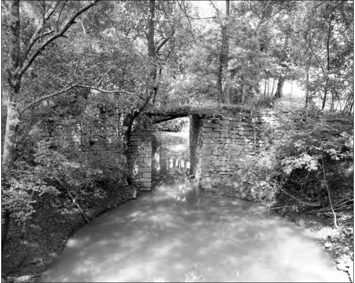
Figure II-03: Bridge at Old Town spanning Brown's Creek on the Natchez Trace, Williamson County (Courtesy of the Tennessee State Library and Archives, Conservation Collection, Bridges, Highways & Roads, Box 10, File 116).
