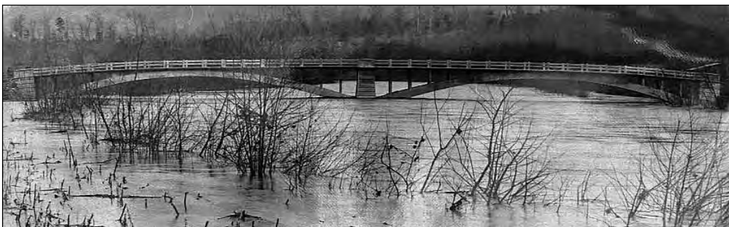
Figure II-59: Three of the bridges demolished as part of the TVA's inundation projects: The Rainbow Bridge in Sullivan County (top); the Walker Ford Bridge over the Clinch River on the Claiborne-Union County line (center); the Nett's (Witt's) Ferry Bridge in Union County during a flood, probably March 1929 (bottom) (Photos from the Steel Collection).
