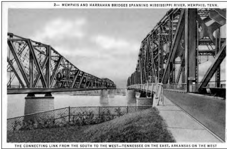
Figure II-07: Historic Postcard showing the Frisco and Harahan Bridges spanning the Mississippi River in Memphis (#14, 79-NonHighway-3 and #77, 79-NonHighway-4). Note the cantilevered roadways on the Harahan Bridge (Author's Collection).
