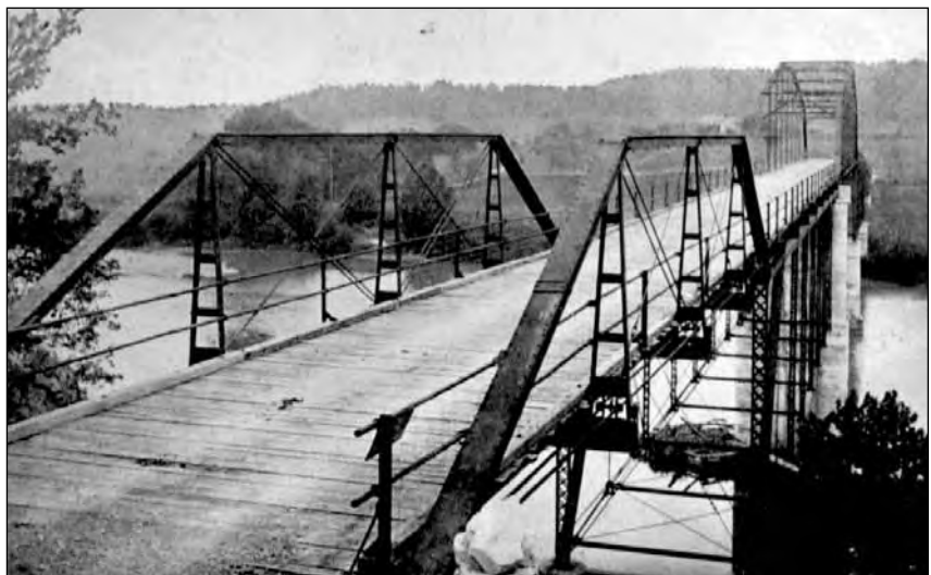
Figure II-60: Truss Bridge at Dandridge, built about 1913 by the Virginia Bridge Company of Roanoke, Virginia. As part of the Douglas Dam project, TVA relocated this bridge to Sevier County where it remained until about 1980. Note the splayed verticals on the pony truss and the combination of pony, through and deck trusses (Courtesy, Tennessee State Library and Archives, LBAT JF013).
