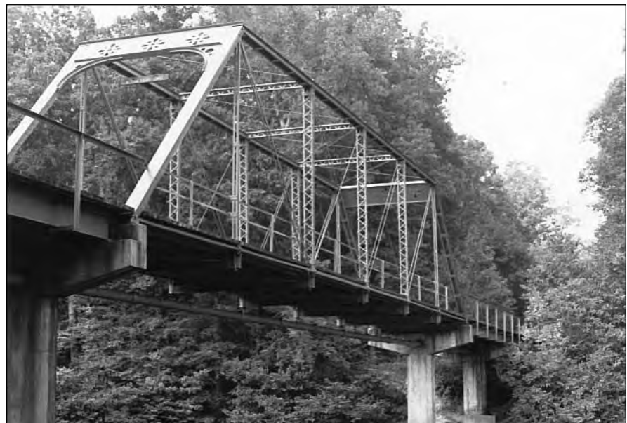
Significant under Criterion C as a representative Pratt truss and as work of the Joliet Bridge Company.
