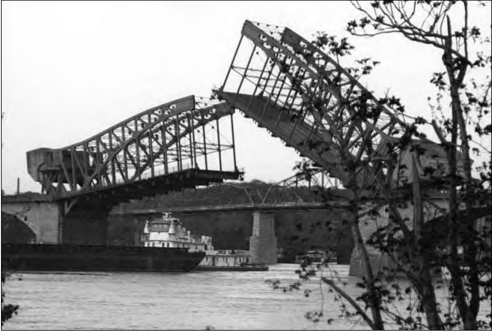
Significant under Criterion A for associations with Dixie Highway and for its role in local politics as well as under Criterion C as rare bascule lift bridge and for concrete arch spans.
