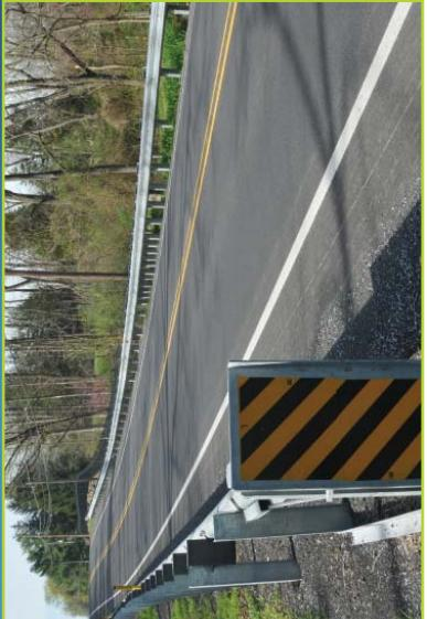
Non energy-absorbing designs do not significantly reduce vehicle speed in a near end-on hit. They are best specified when there is a long, clear, traversable area behind them parallel to the guardrail installation, such as one often found in a flat freeway median. Crash-testing has shown this runout distance can exceed 150 feet. Therefore, barrier installations less than 150 feet in advance of any shielded object should be introduced with an energy-absorbing terminal design.
