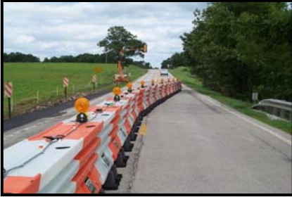
Internal Steel Frame
