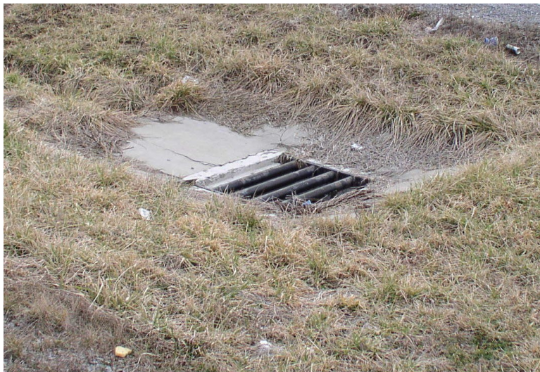
Figure 7-4 Typical Median Ditch Inlet
