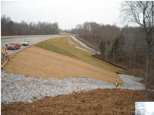
Low point in roadway required both toe ditches to be stabilized with rip rap
