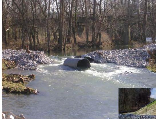
After the water receded. The contractor had to remove stone from creek channel by hand.
