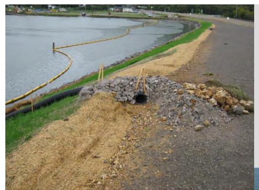
Multiple slope drains added to convey surface runoff to toe of slope until roadway is completed (change order to construction)
