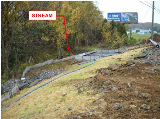
No construction easement or enough stream buffer provided for sediment filter bag.
