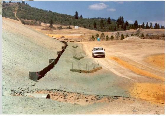
Silt fence shouldn't be depicted perpendicular to contours. No outlet provided at low point in silt fence at toe of slope resulting in silt fence being overtopped during storm event
