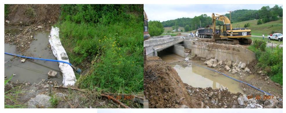
Stream diversion using bypass pumpingundersized?
