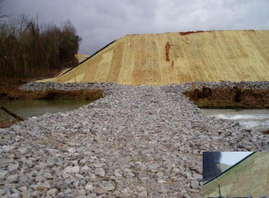
Temporary stream crossing – installed correctly?
