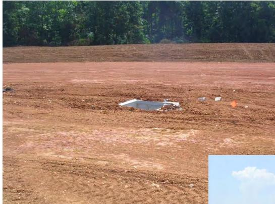
Inlet protection is considered a perimeter control because the discharge from area drains and curb inlets is usually at the project boundaries
