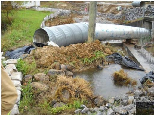
Suspended pipe diversion on box culvert extension on inlet – not properly diverted into inlet for high flows
