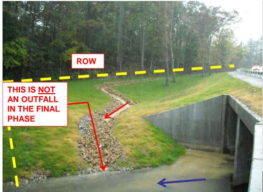
Relocated stream channel discharging to another stream
