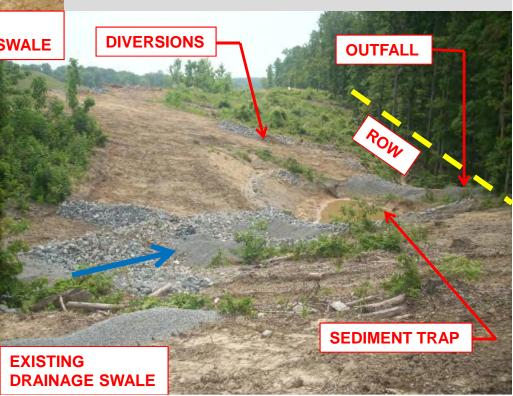
Multiple culverts discharging into a wet weather conveyance
