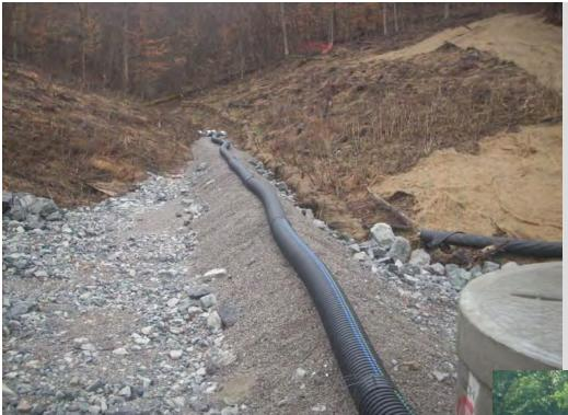
Stream diversion for channel relocation – plastic pipe and gravel berm
