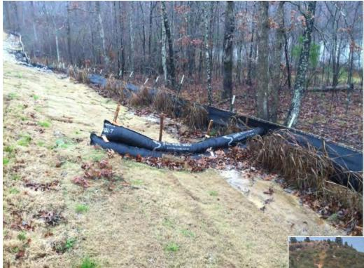
Silt fence using erosion eels for J-hooks on silt fence not placed on contour
