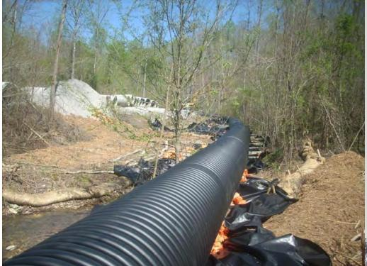
Suspended pipe stream diversion – pipe size provided on EPSC plans
