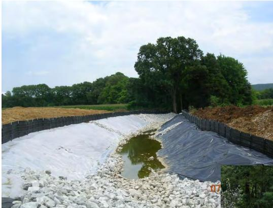
Temporary stream diversion and crossing to construct a box culvert.
