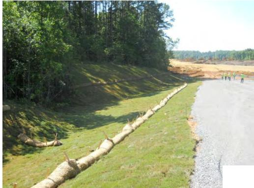
Sediment tubes used to protect a roadside ditch slopes until the sod is rooted.
