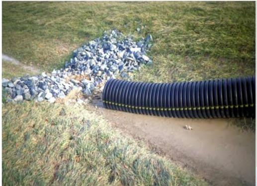
Check dams used as slope drain outlet protection and runoff control within ditch
