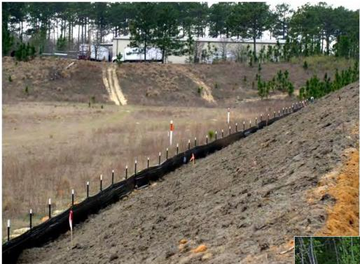
Silt fence placed at toe of slope = no sediment storage and hard to perform maintenance and removal
