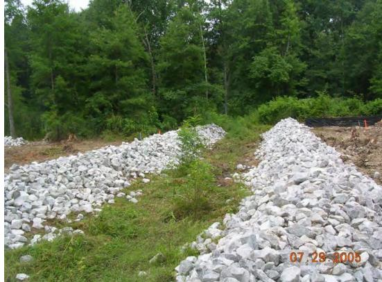
Rip-rap berm used to protect an intermittent stream.
