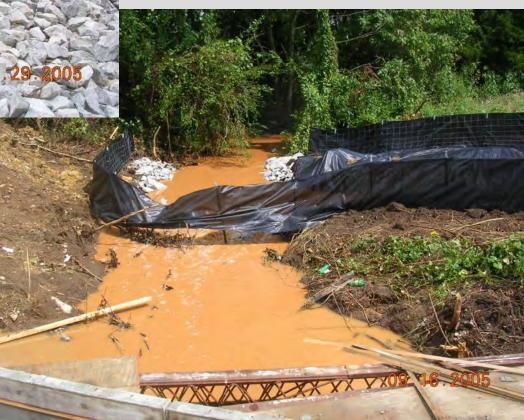
Verify that the channel lining specified in the stream diversion can handle the velocities during the design storm event.
