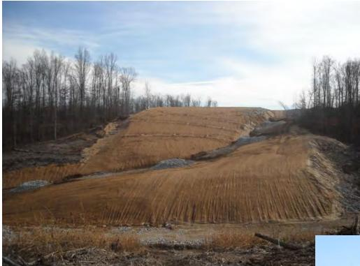
Diversion ditches and matting used to protect steep slope areas during construction (intermediate EPSC phase)
