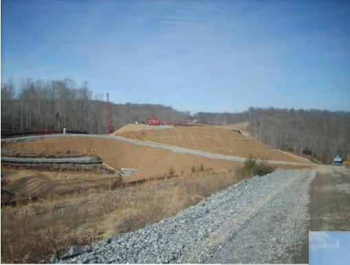
Bridge abutment slopes protected with sediment tubes and matting (intermediate EPSC phase)
