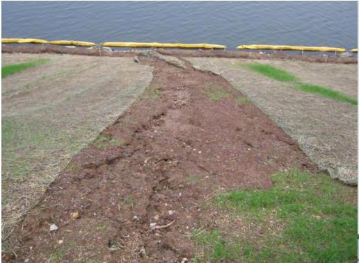
No slope drains depicted in EPSC plans. Several slope failures occurred due to surface runoff from compacted roadway surface
