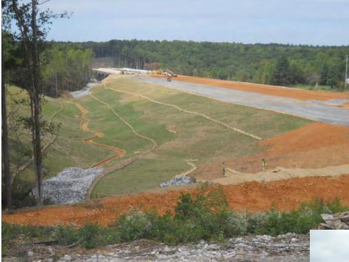
Sediment tubes placed on slopes to break up surface runoff into to relocated stream channel (final EPSC phase)
