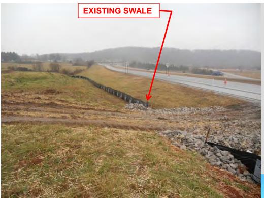
No temporary pipe culvert included for existing drainage swale
