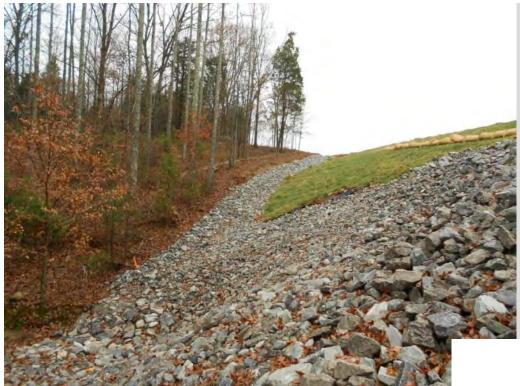
Typically toe ditches are on a very steep gradient and need stabilization
