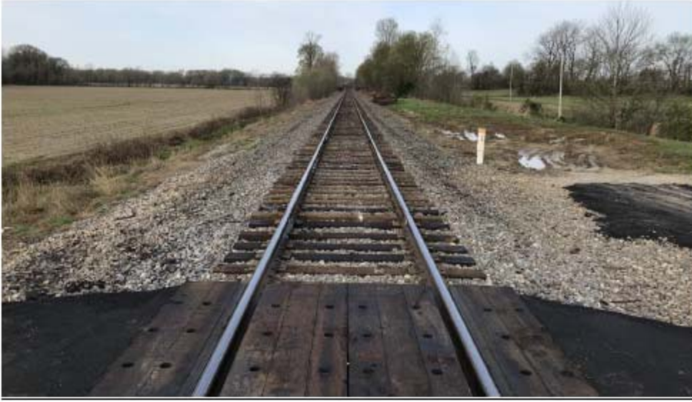
LOOKING WEST ALONG THE CROSSING 297413R
