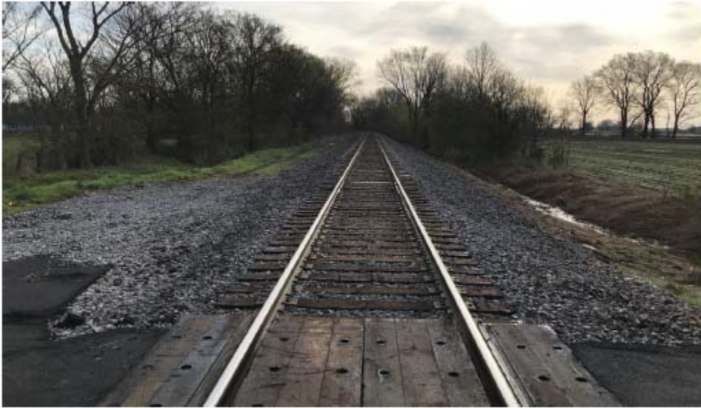
LOOKING EAST ALONG THE CROSSING 297413R
