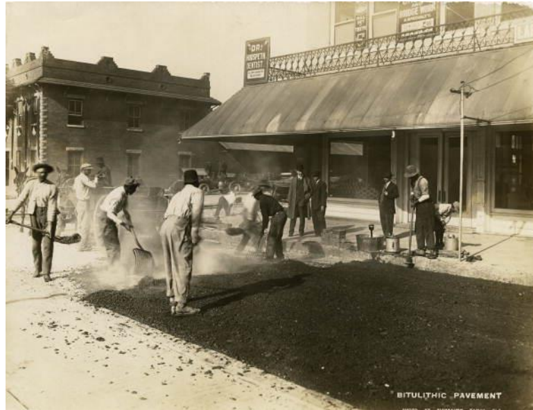
Figure 2-1. Bitulithic pavement placement process. Tampa, Florida (1920s.)
