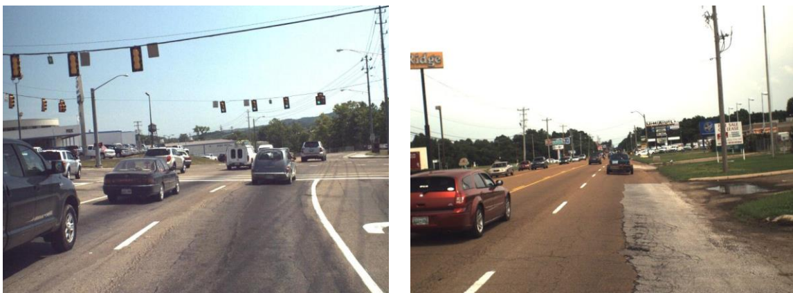
Figure 12 Typical “poor” pavement sections with both low PSI and high rutting depth
