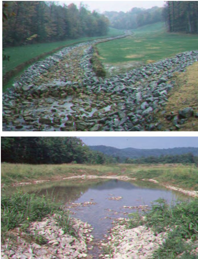
Figure 4.1. Example photos of an open limestone channel (top) and a vertical flow wetlands (bottom). Photos from Paul Ziemkiewicz, West Virginia University, 2002.
