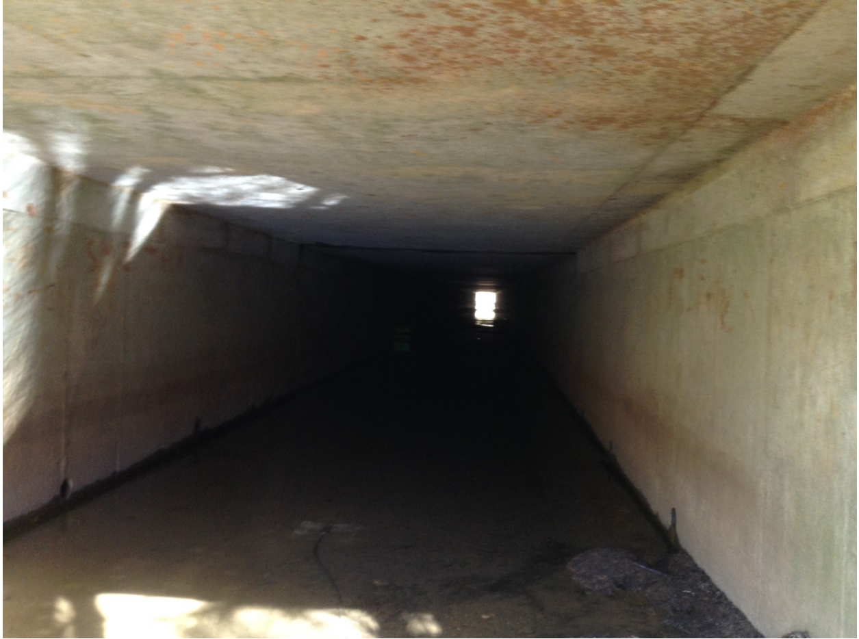
Figure B.3. Site SC1 sampling point looking upstream through conveyance tunnel.
