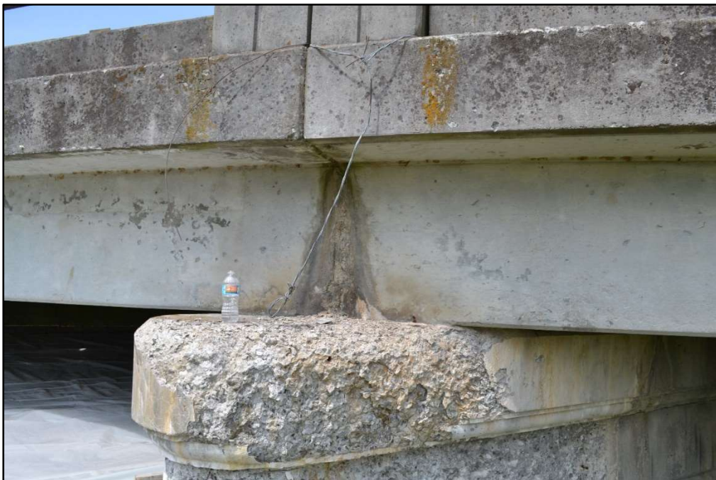
Figure 4-6: Substructure – Deterioration
