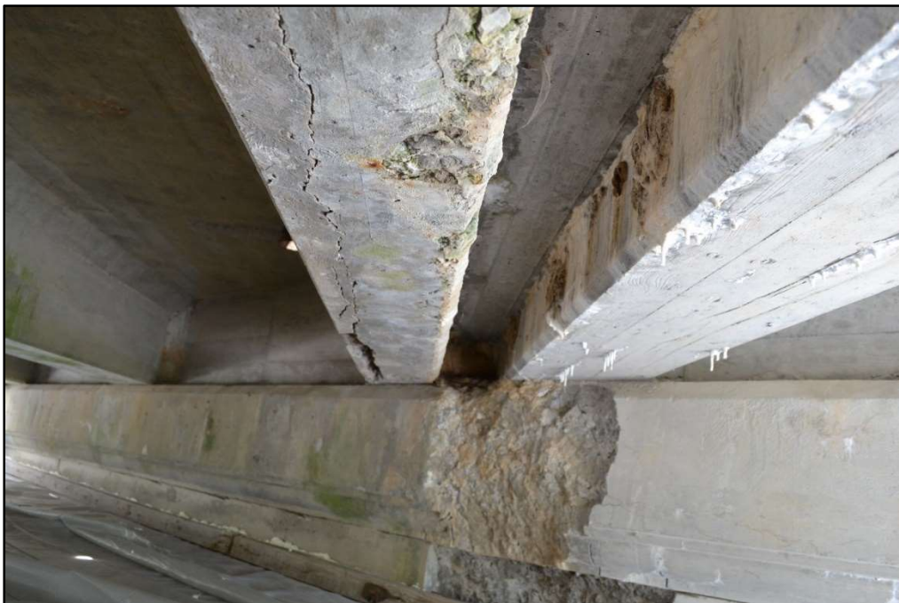
Figure 4-18: Superstructure - Deterioration
