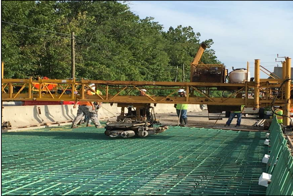
Figure 4-39: Deck – Concrete Placing
