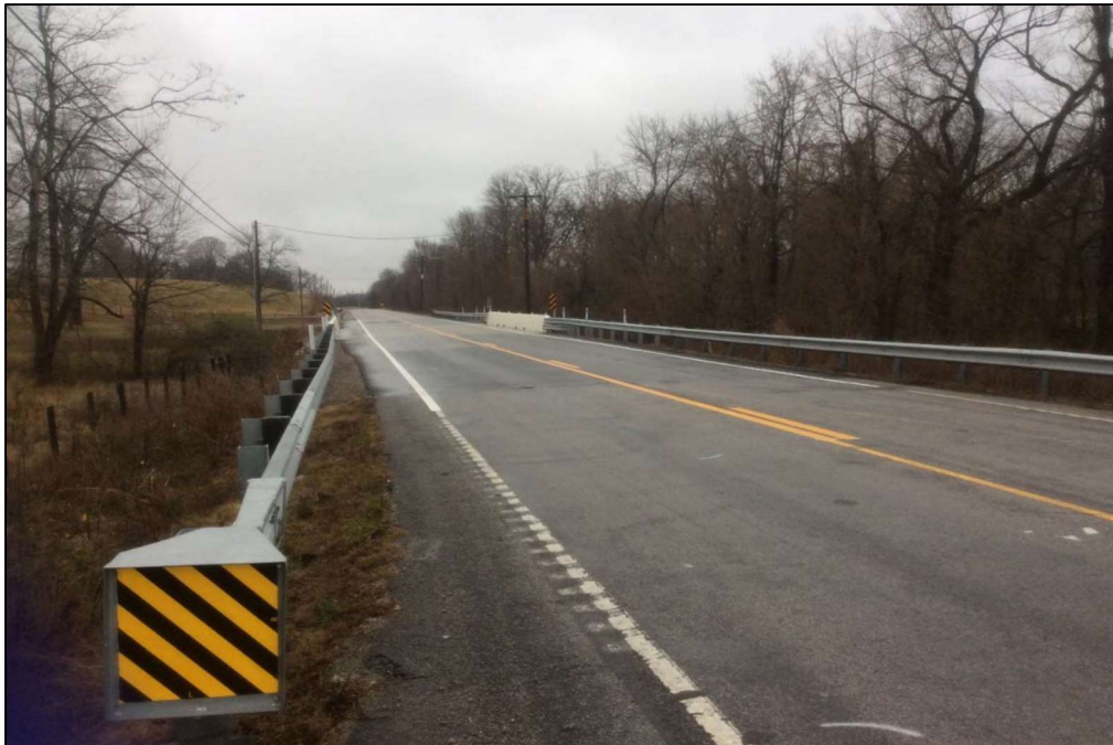
Figure 4-56: Completed Deck – Bridge No. 94-SR11-0.87
