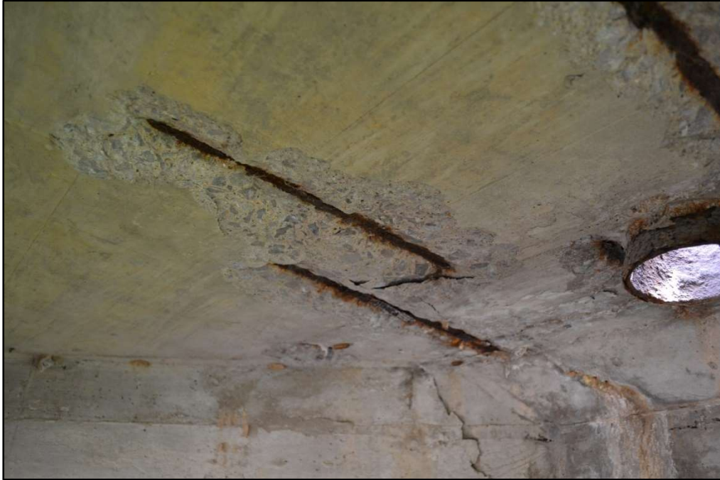
Figure 4-29: Deck - Deterioration
