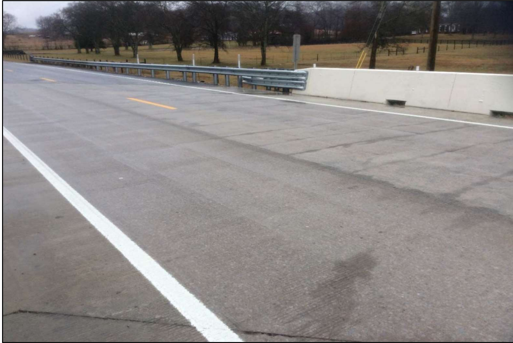
Figure 4-51: Completed Deck – Bridge No. 94-SR11-0.59
