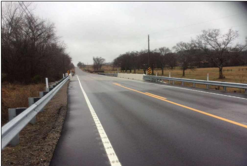
Figure 4-44: Completed Deck – Bridge No. 94-SR11-0.59
