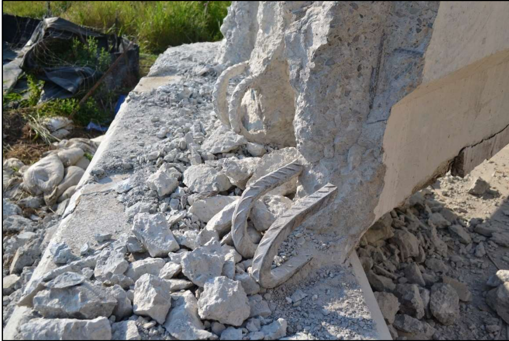
Figure 4-23: Superstructure – Good Condition Without Corrosion
