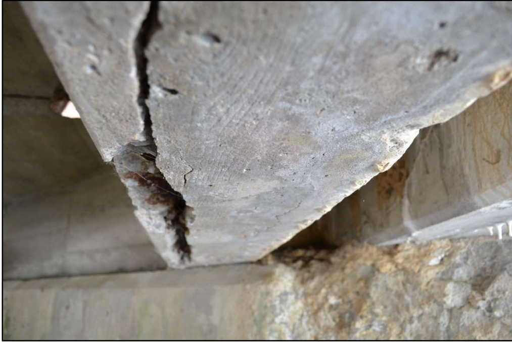
Figure 4-19: Superstructure - Deterioration
