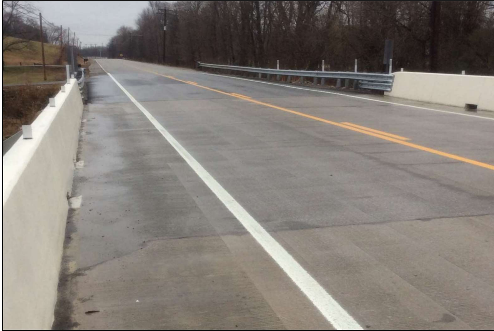
Figure 4-59: Completed Deck – Bridge No. 94-SR11-0.87
