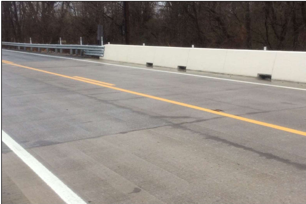
Figure 4-58: Completed Deck – Bridge No. 94-SR11-0.87
