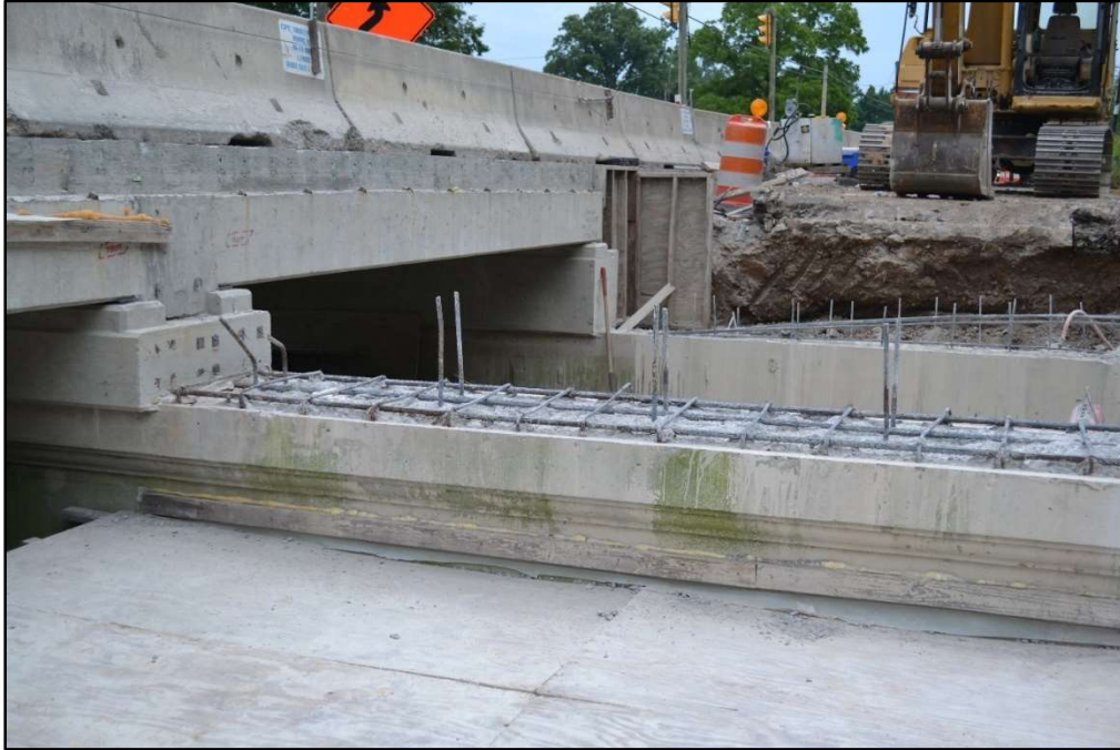
Figure 4-11: Substructure – Prepared for Modification
