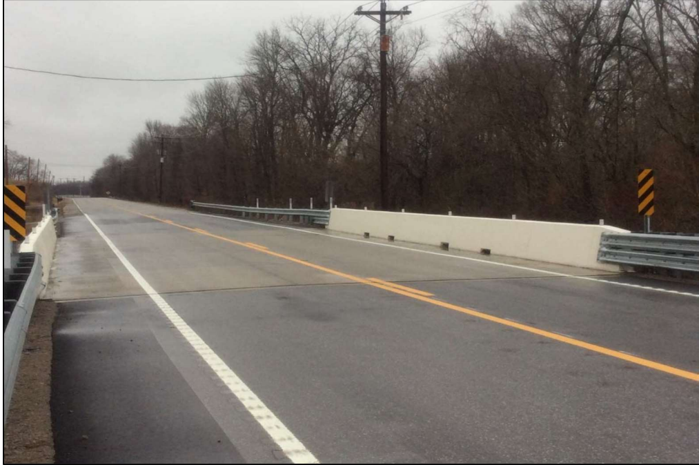
Figure 4-57: Completed Deck – Bridge No. 94-SR11-0.87
