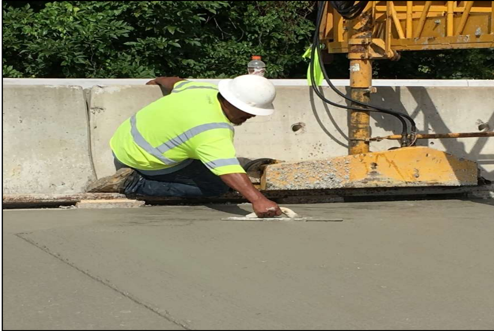
Figure 4-43: Deck – Concrete Placing
