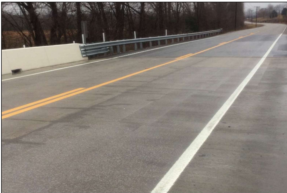
Figure 4-62: Completed Deck – Bridge No. 94-SR11-0.87
