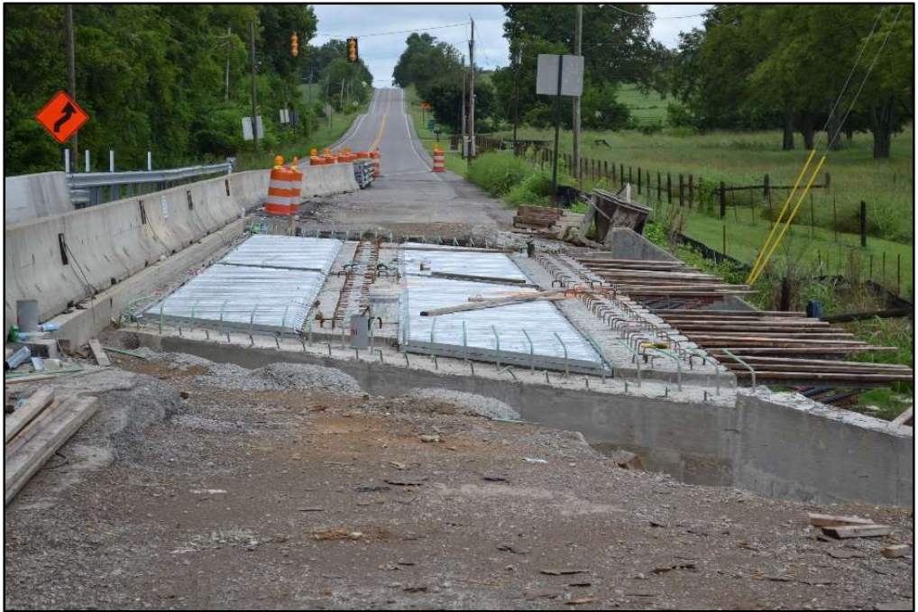
Figure 4-36: Deck – Form Installation
