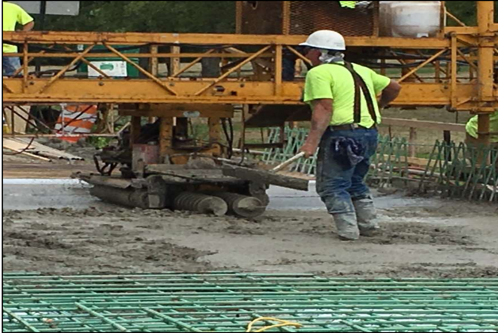
Figure 4-41: Deck – Concrete Placing
