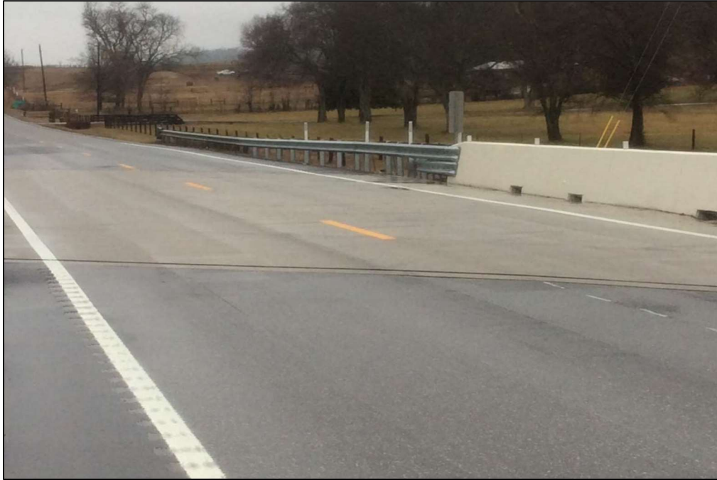
Figure 4-47: Completed Deck – Bridge No. 94-SR11-0.59
