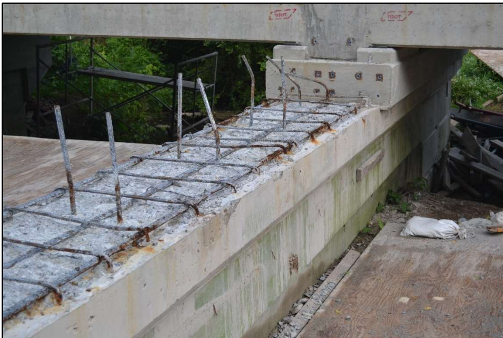
Figure 4-12: Substructure – Prepared for Modification
