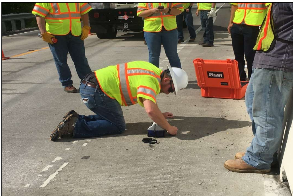
Figure 5-40: Locating Reinforcing Steel
