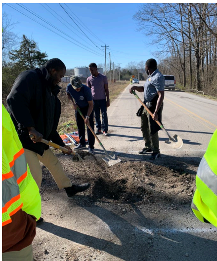
(a) Reclaiming Pavement Materials
