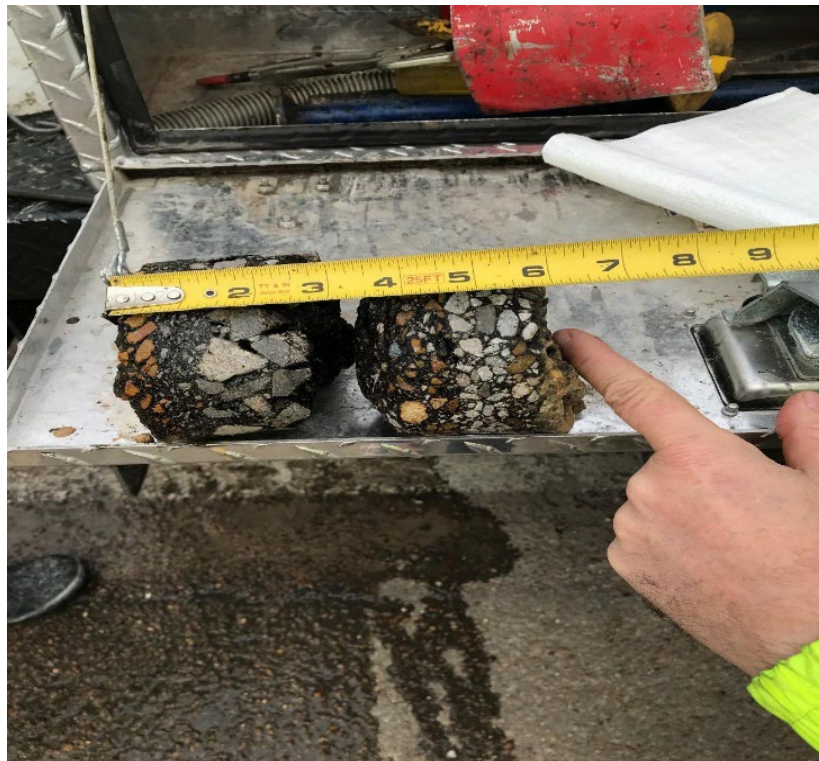
Figure C 6 Core#8 (6 1/4") Hole depth 9"-lost 2 3/4"
