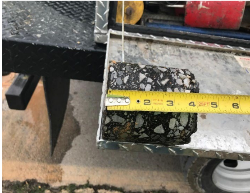
Figure C 1 Core#3 (4") was drilled at 1.1 mile and corresponds to Sample # 2
