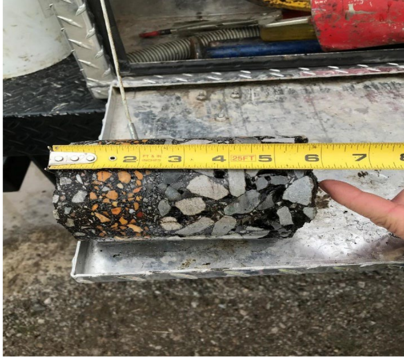
Figure C 5 Core#7 (6") was drilled at 3.1 mile and corresponds to sample # 4
