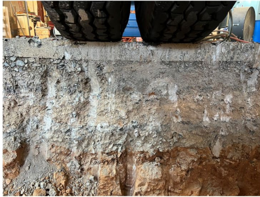
Figure 4-26. Trench cut in the three lanes (a) Inverted pavement 1, (b) Inverted pavement 2, (3) Inverted pavement 3
