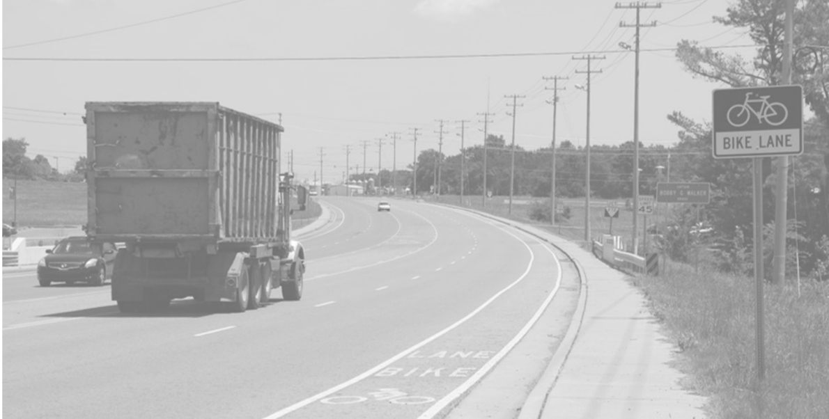
Lewisburg's Ellington Parkway has two lanes in each direction with a center turn lane to accommodate a high volume of vehicles while providing efficient cross-county travel
