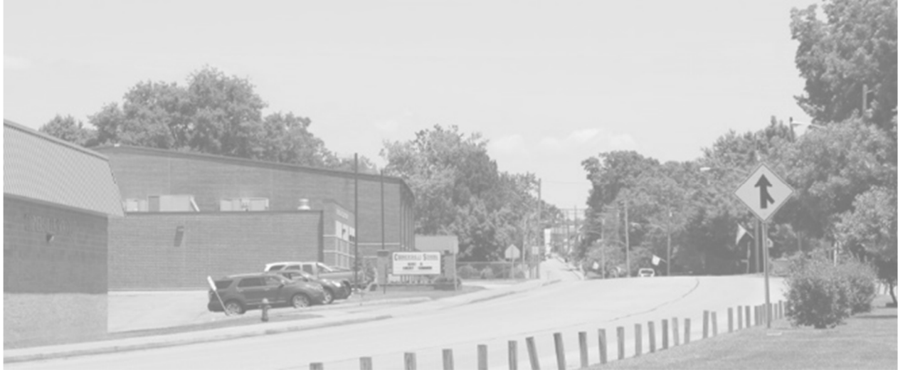
Cornersville's Middle and High School is located along S. Main Street (US-31A)
