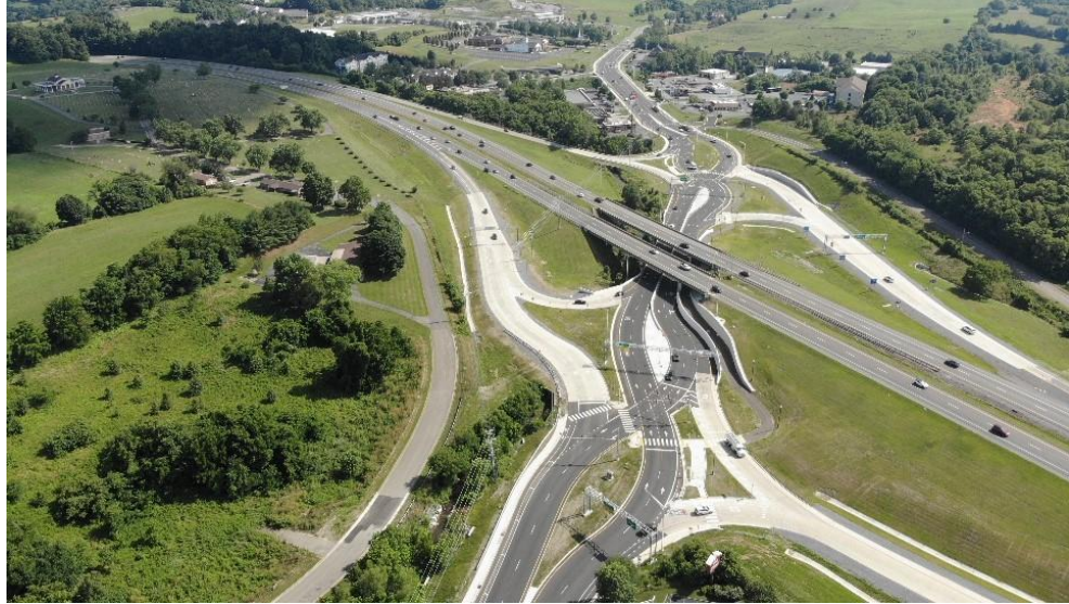
Figure 32. Newly Constructed Diverging Diamond Interchange on I-26 at Exit 17
