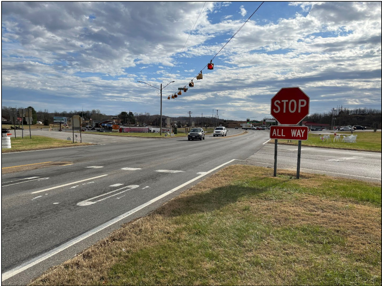
Figure 2-3. Intersection of Austin Peay Highway and Highway 31-E (looking south)
