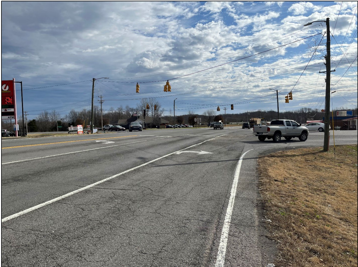
Figure 2-6. Intersection of Highway 31-E and SR 52 (looking south)
