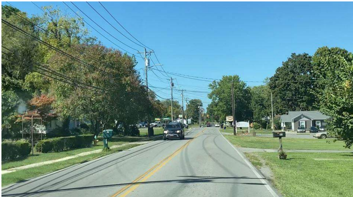
FIGURE 4: PHOTO OF TYPICAL SECTION
