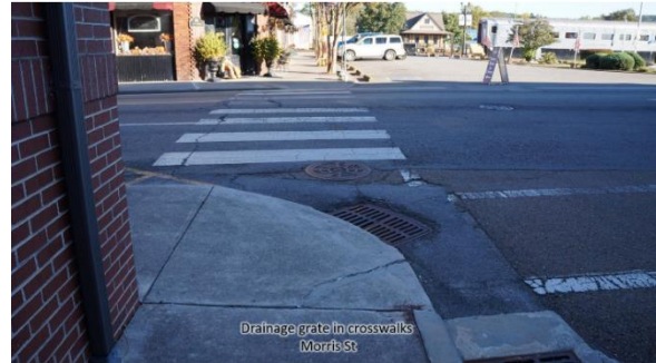
Figure 22: Drainage at Morris Street
