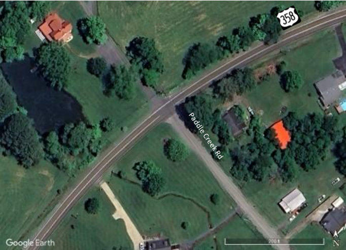
Figure 2-14 Paddle Creek Road Aerial View
