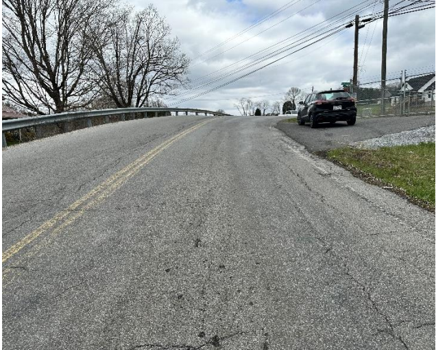
Figure 2-17 Driver View Approaching Intersection From Pleasant Grove Road
