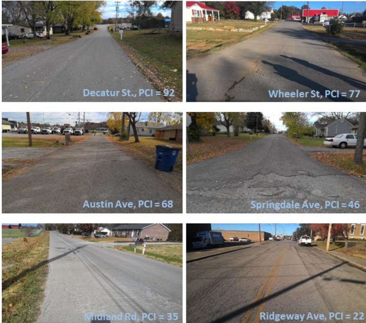
Figure 5. Pavement images with different PCI values.
