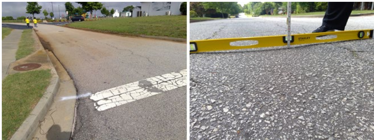
Figure 3. Example of pavement condition data collection and distress measurement.
