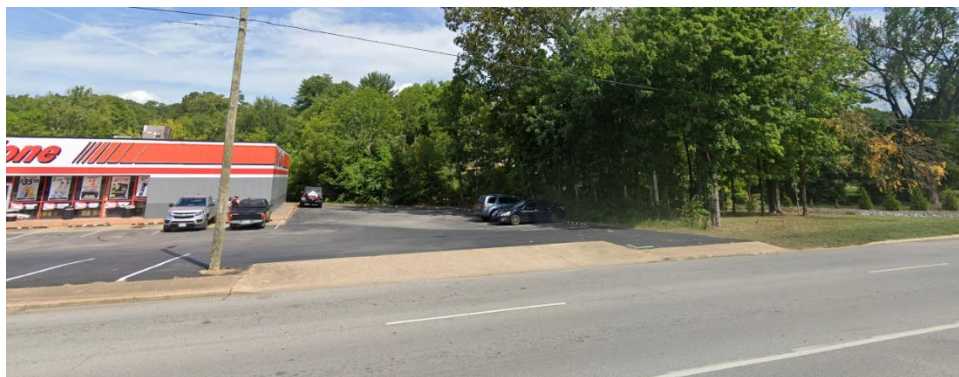
Figure 26: Dayton Boulevard at Newberry Street - Sidewalk Abruptly Ends
