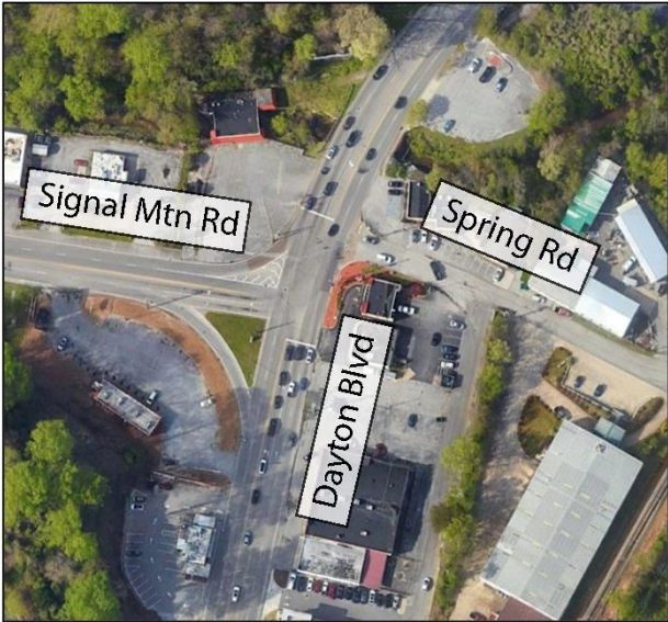
Figure 34: Dayton Boulevard at Signal Mountain Road
