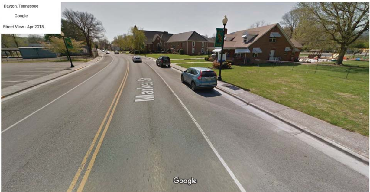
Figure 19: Market St., between Hickory St. and California Ave., across from the Dayton Youth Baseball Complex. Image taken facing southwest. Approx. 8 ft paved shoulder being used for parking. Image capture: Apr 2018 © 2022 Google
