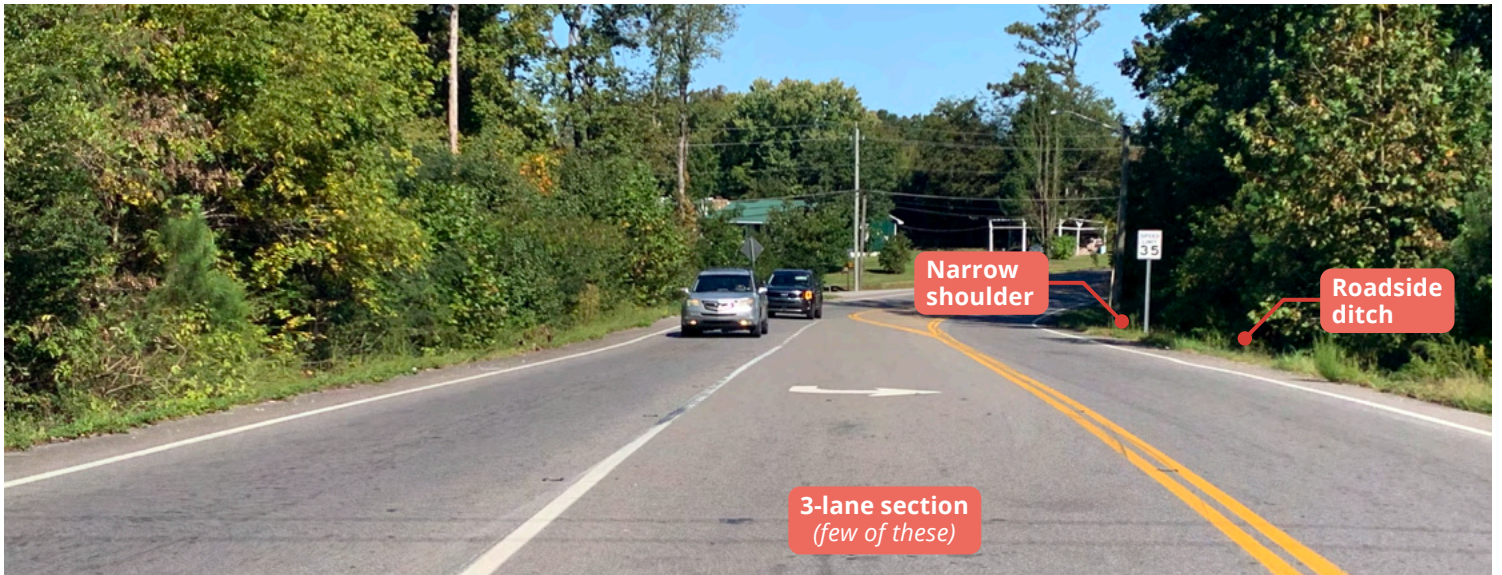
Michigan Avenue Road intersection with Benton Pike, looking northwest.
