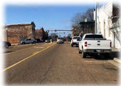
Highway 64 (SR-15) looking west Between Water Street and Main Street
