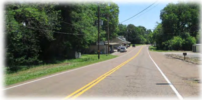
Highway 64 (SR-15) looking east East of 3 rd Street
