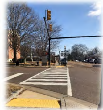
Crosswalk on North Leg
