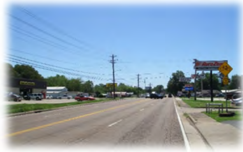
Highway 64 (SR-15) between Tennessee St. and Tate St.
