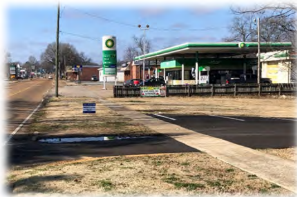
Sidewalks on Highway 64 (SR-15) East of Lauderdale Street
