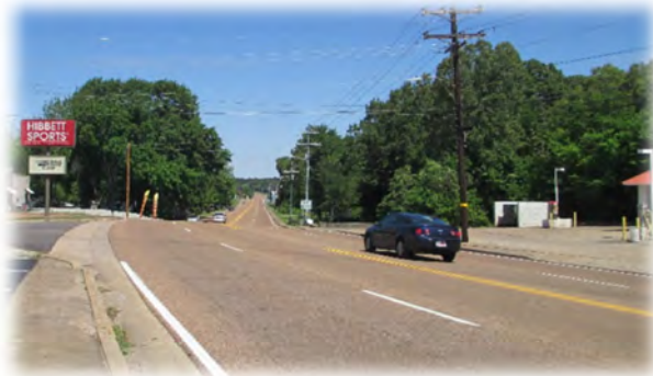
Highway 64 (SR-15) West of Porter Street
