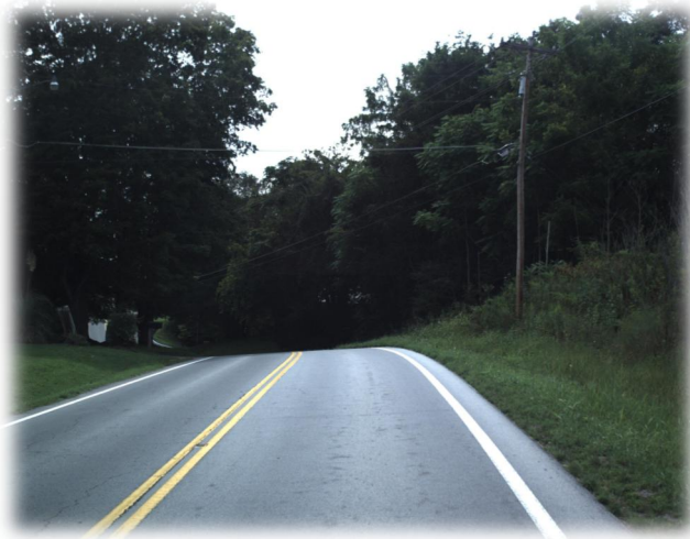
SR-49E, APPROACHING OLD HIGHWAY 47
