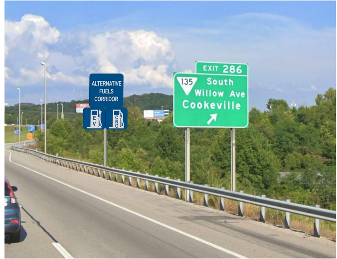
Illustration of Corridor-Ready MUTCD Signage along I-40.
