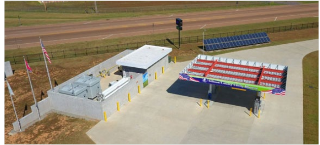
Gibson County Utility District's first CNG refueling station in Trenton, TN. Photo: Gibson County Utility District
