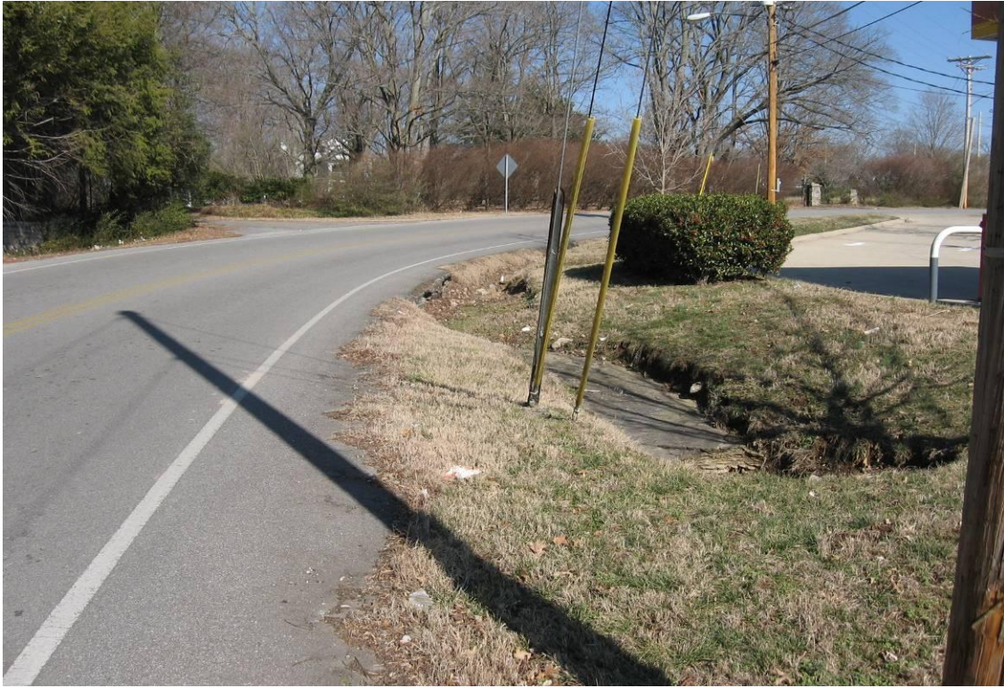
Looking North along Halltown Road at concrete drainage ditch
