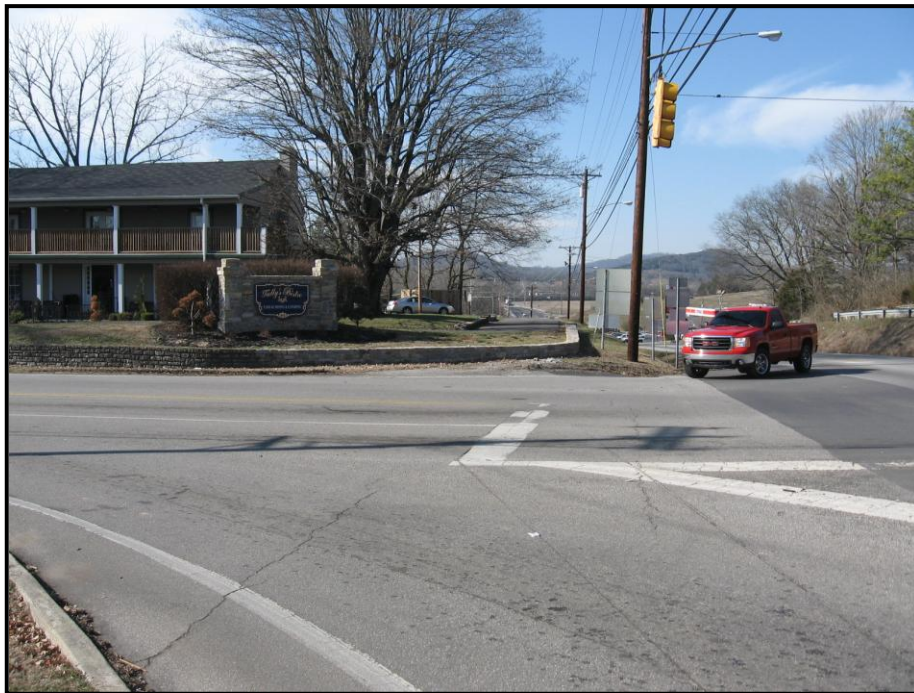
Photo 7 - Line of Sight issues for SR-141 channelized right turn
