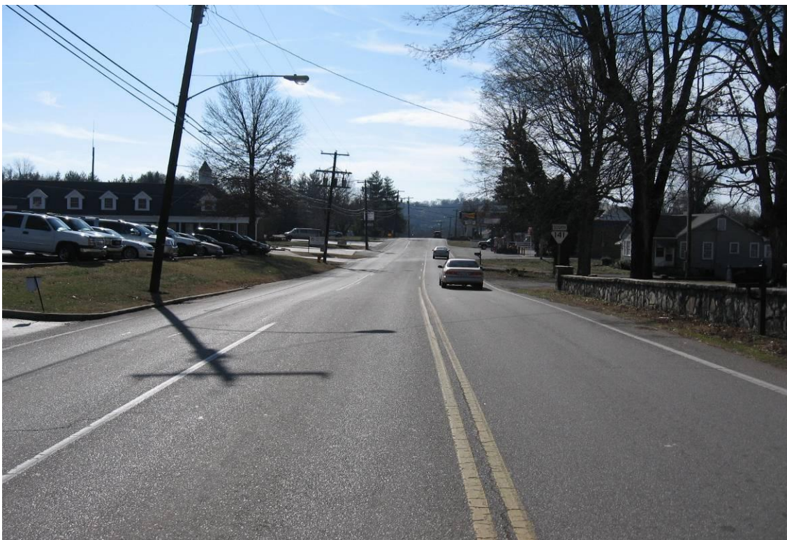
Looking South along SR-141 (South of the Intersection)
