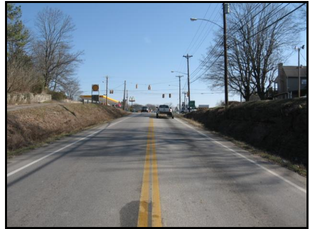
Photo 2 - SR 10/25 Eastbound Approach
