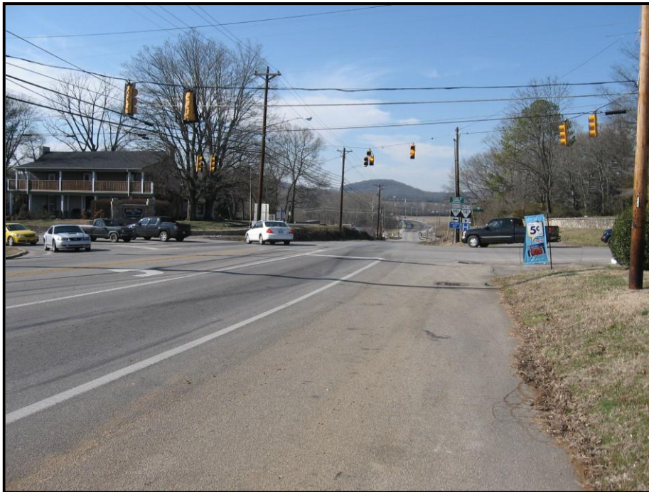
Photo 8 - Lack of glare protection on westbound signal heads
