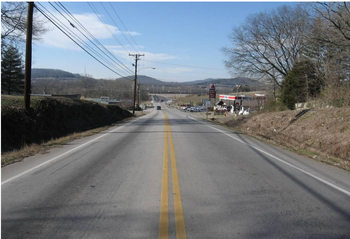
Looking West along SR 10/25 (West of Intersection)
