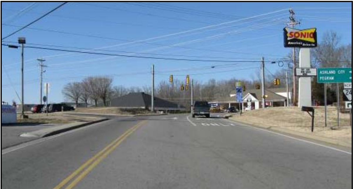
View north along SR 249/Luyben Hills Road toward Intersection with Kingston Springs Road
