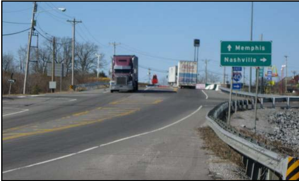
View north from south side of I-40/SR 249 Interchange
