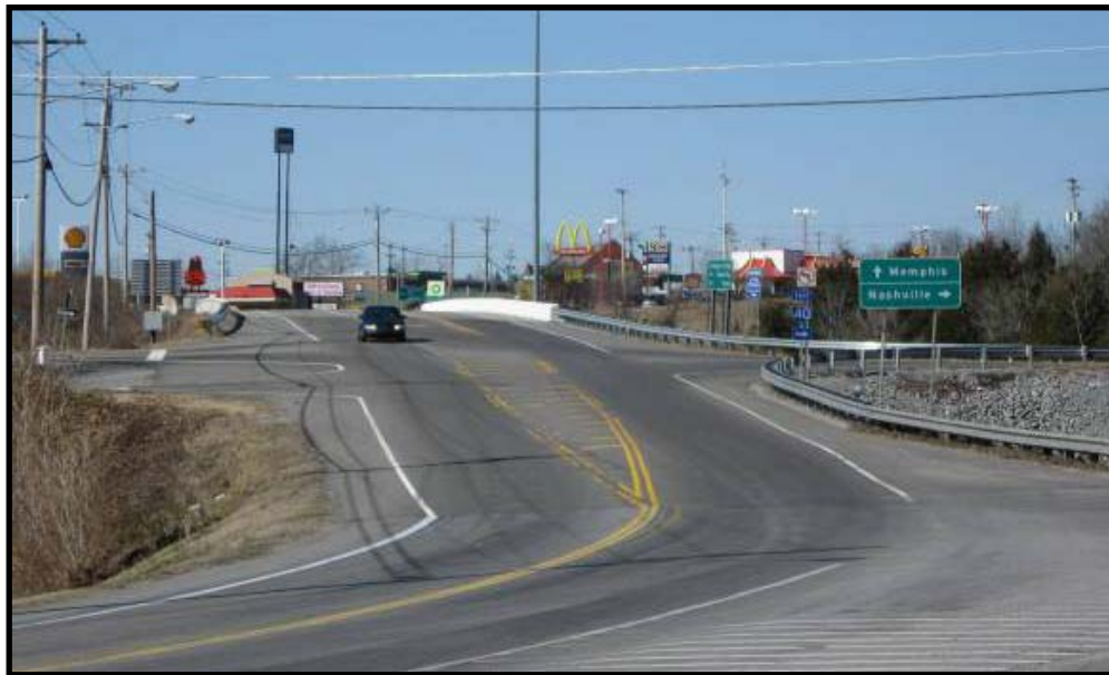
View north of I-40/SR 249 Interchange
