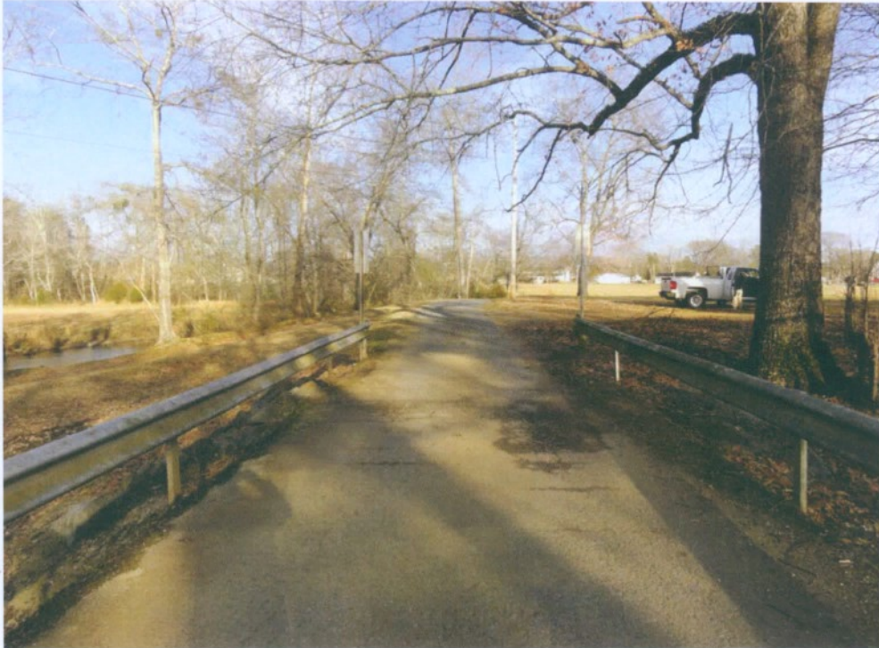
Bridge Looking East on West 2 nd Street
