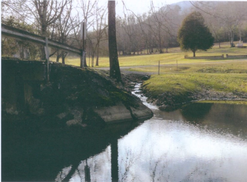
Slope Repair West Approach
