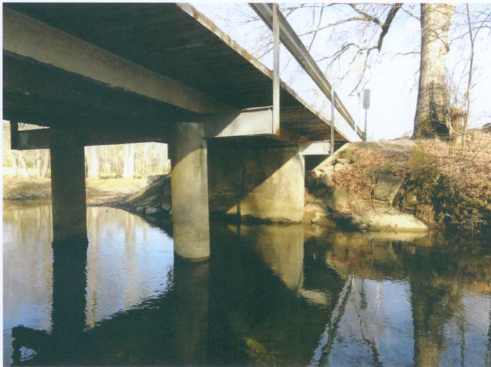
Substructure Looking East
