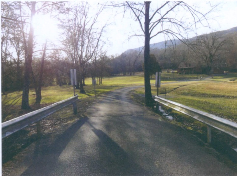
Bridge Looking West on West 2 nd Street
