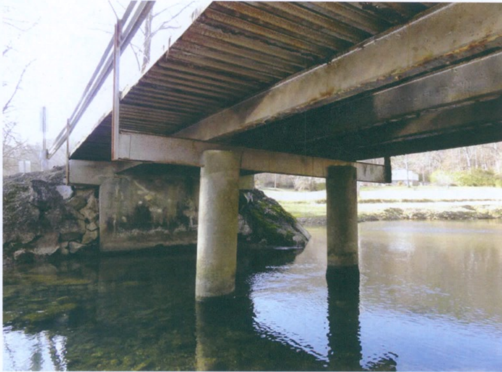
Substructure Looking West
