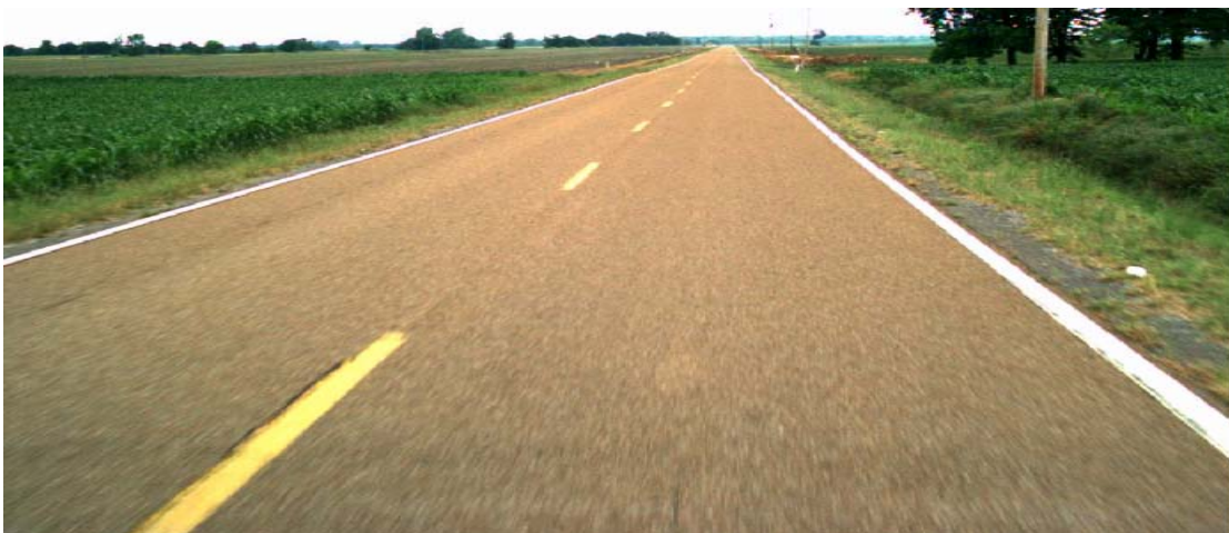
Existing State Route 22 10' travel lanes with 4' shoulders
