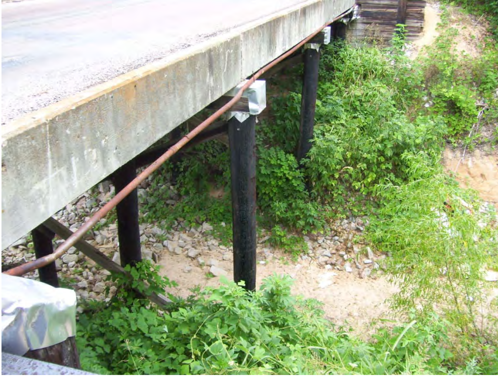
View of bridge inlet.
