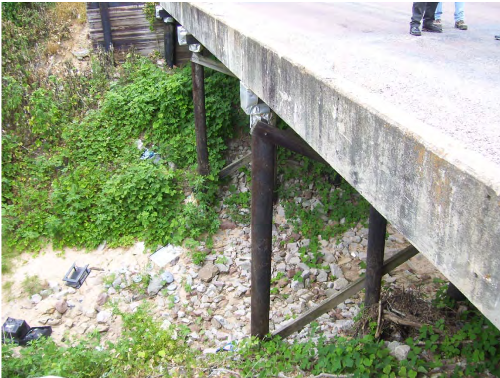
View of bridge outlet.
