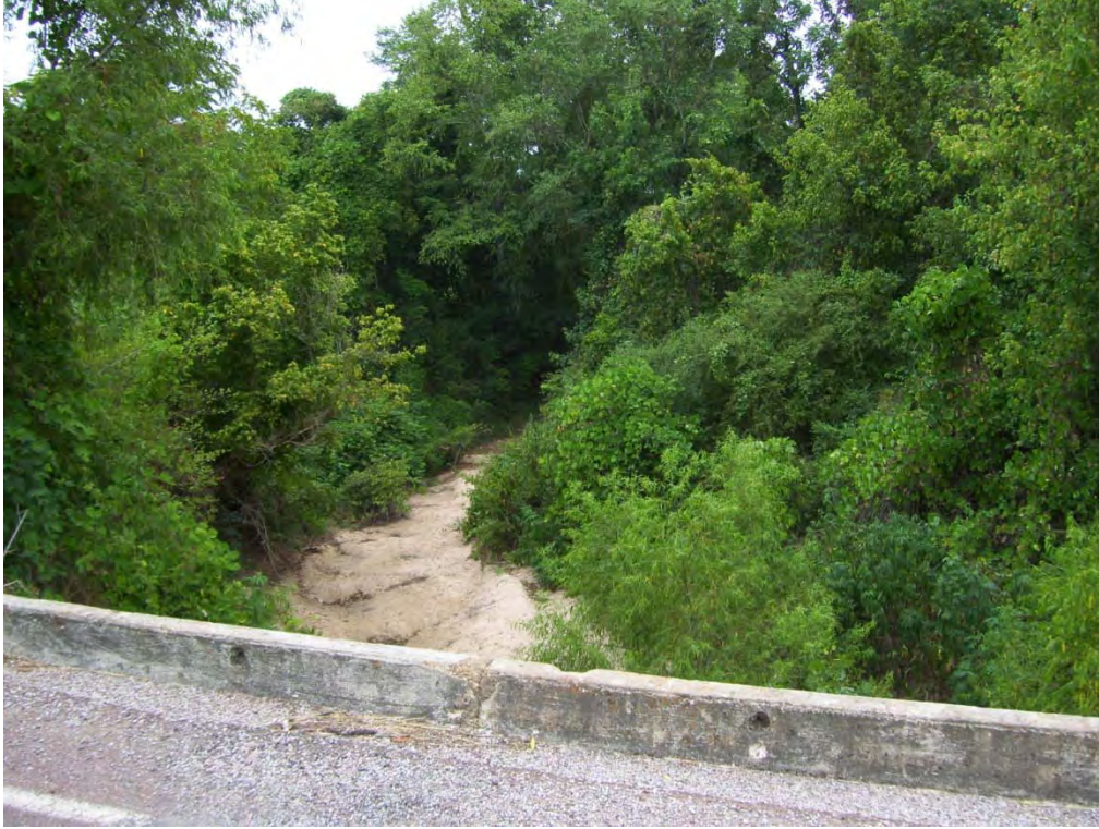
View upstream from bridge.
