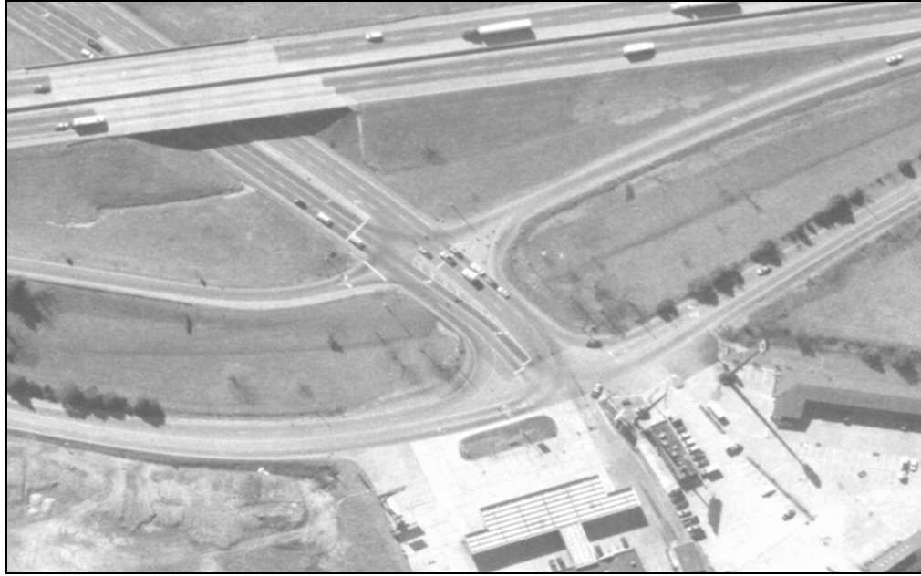
Photo 5: Aerial view of I-75 at Hunter Road & Mountain View Road
