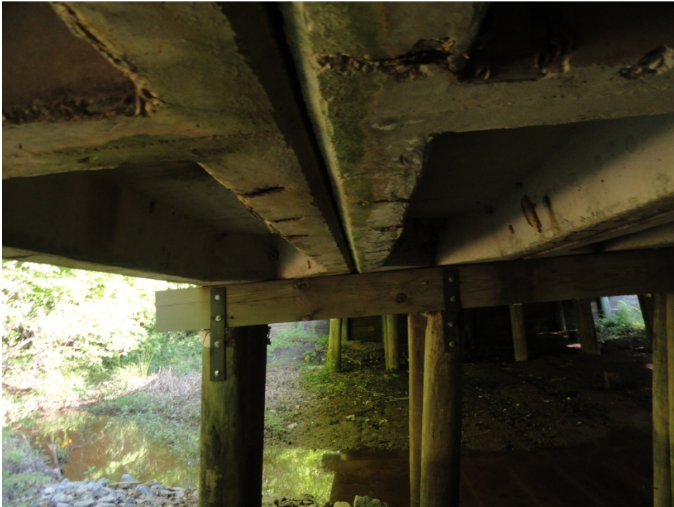
Bridge Deck and Piers
