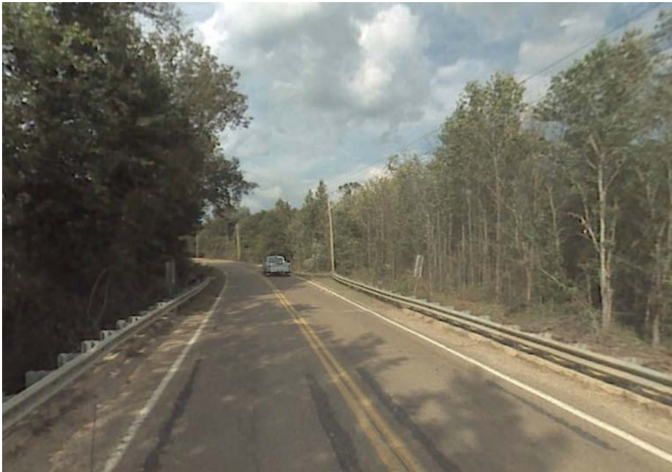
Southbound Approach – Looking North
