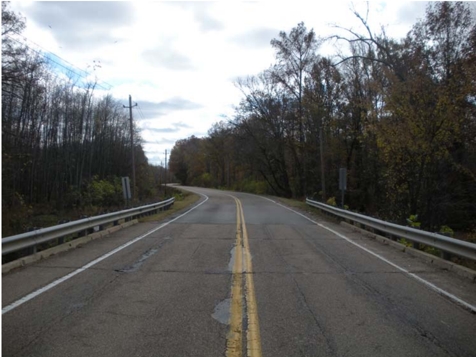
Northbound Approach (Looking South)
