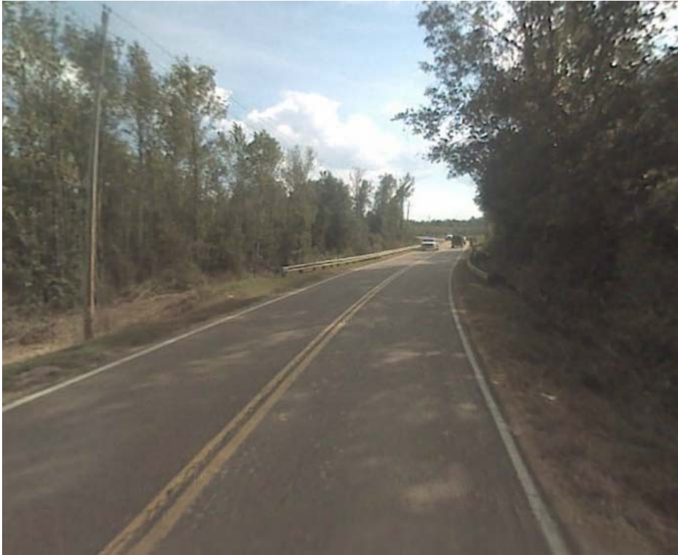
Southbound Approach – Looking South
