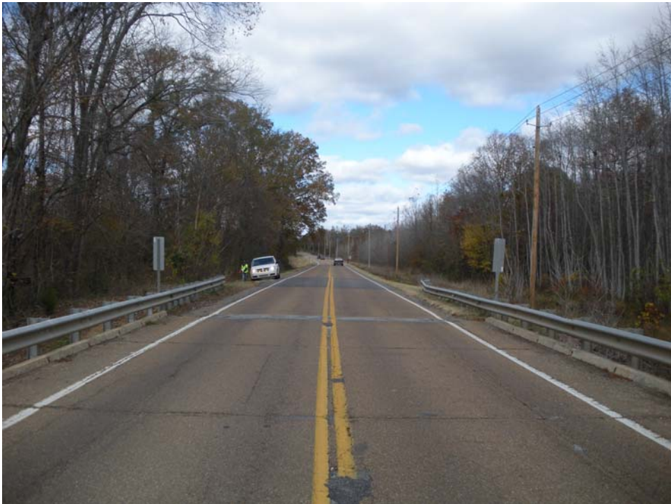
Southbound Approach (Looking North)
