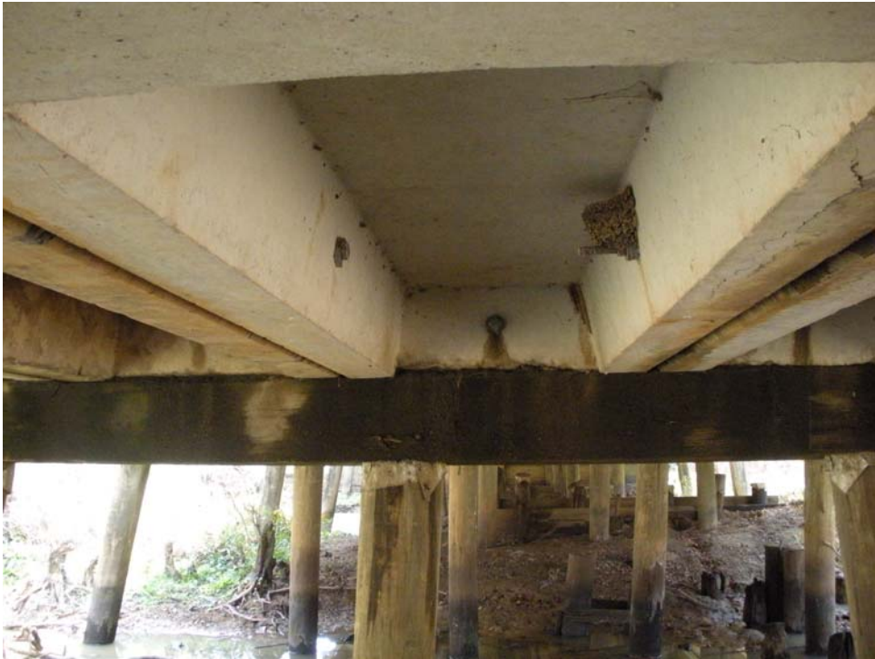
Concrete Channel Sections with Timber Substructures
