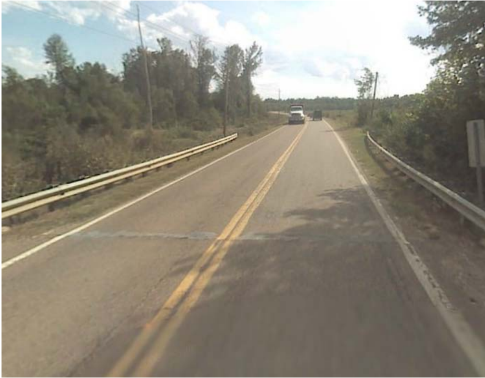
Northbound Approach – Looking South
