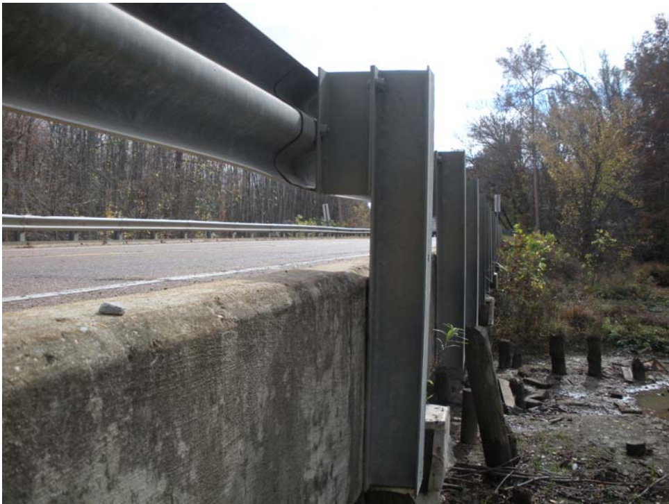
Guardrail Mounted to Bridge
