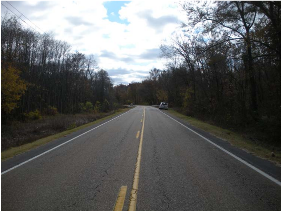
Southbound Approach (Looking South)
