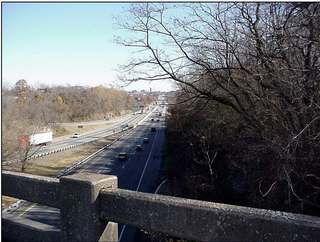
Photo 6: Proposed ramp location (Spence Lane to I-40 Eastbound)
