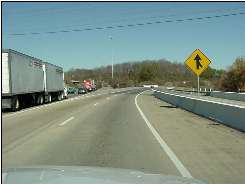
Photo 4: I-24 to I-40 with EB Murfreesboro Road Entrance Ramp
