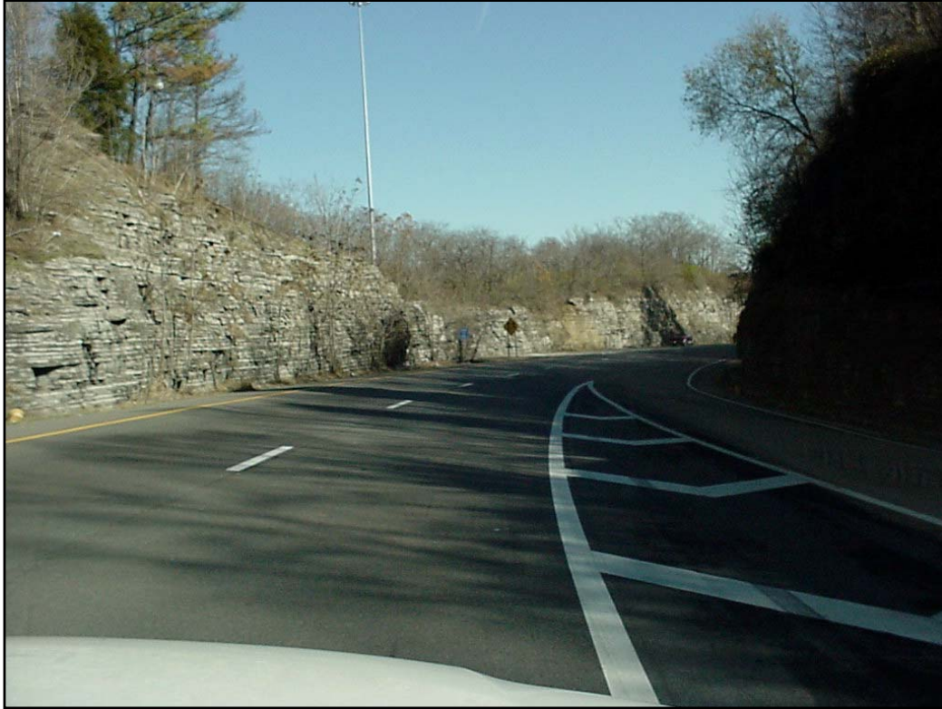
Photo 5: I-24 to I-40 with WB Mufreesboro Road Entrance Ramp
