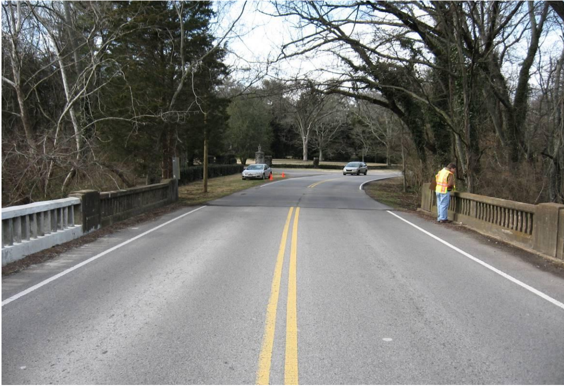
Looking Northwest from Bridge
