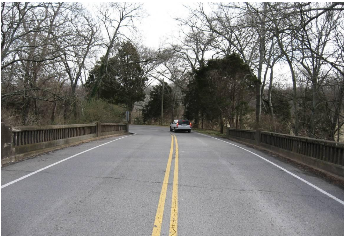
Looking Southeast from Bridge
