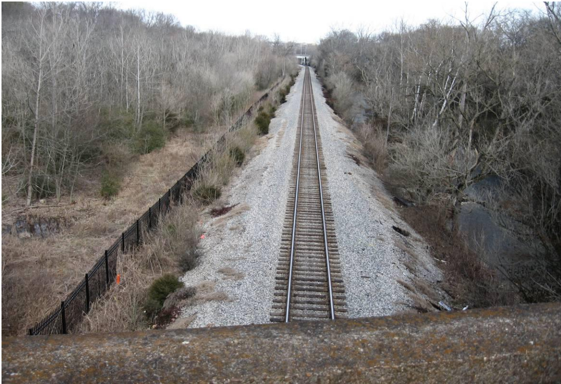
Looking Northeast along CSX Railroad from Bridge
