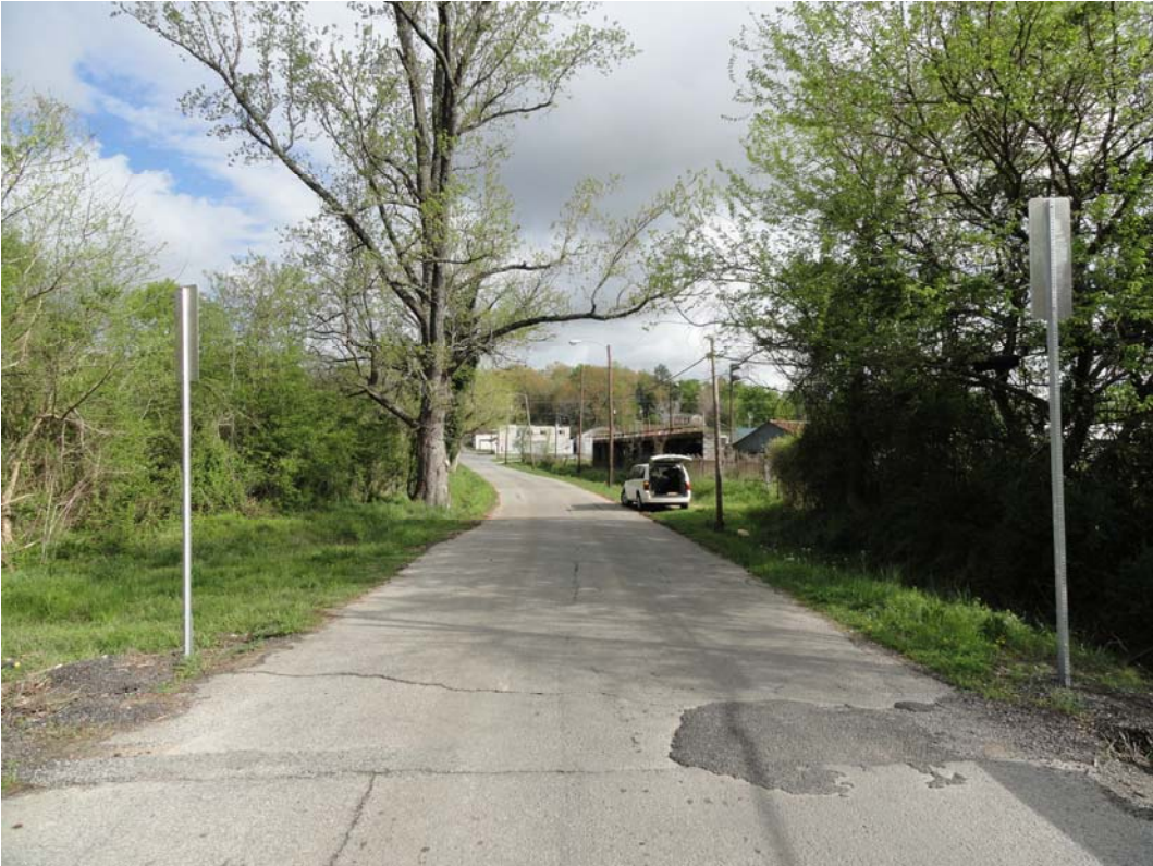
Bridge Looking North on Fern Avenue
