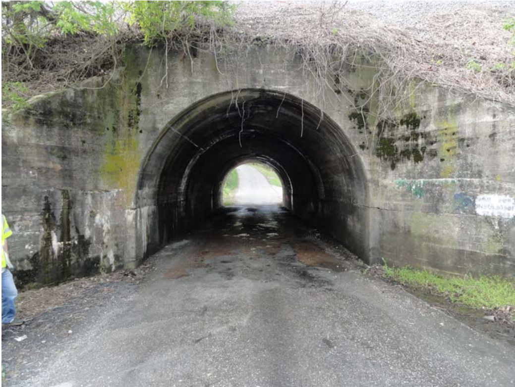
Bridge Looking South on Fern Avenue
