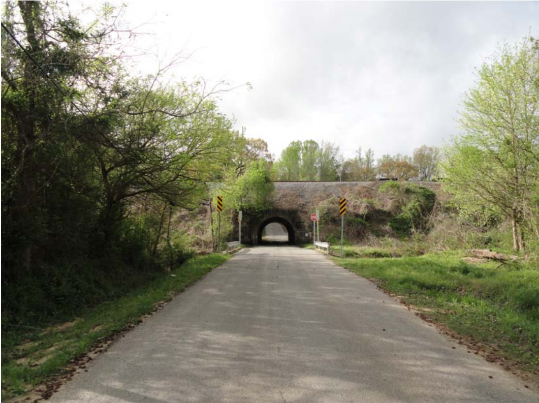
Southbound Bridge Approach on Fern Avenue
