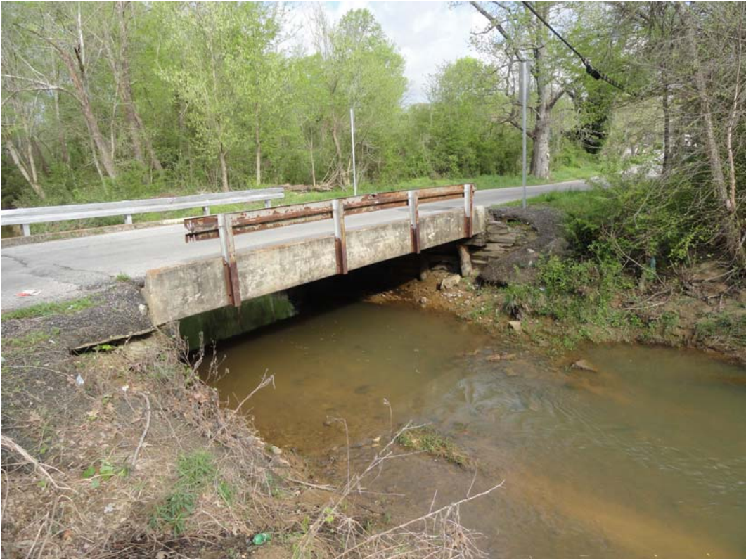
View of Structure
