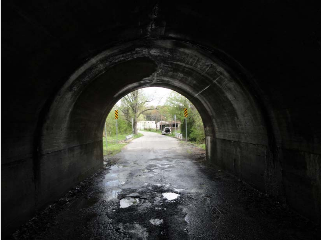
Northbound Bridge Approach on Fern Avenue
