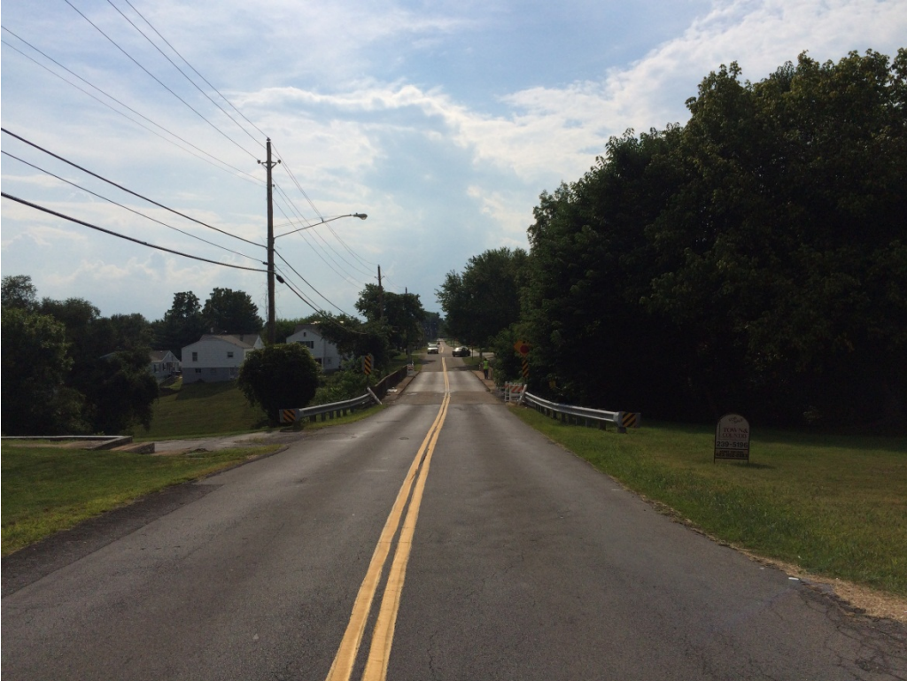
Westbound Bridge Approach on Local Route 03899
