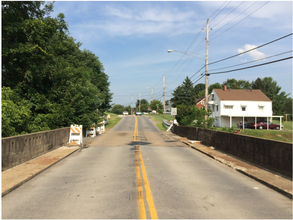
Center of Bridge Looking East on Local Route 03899
