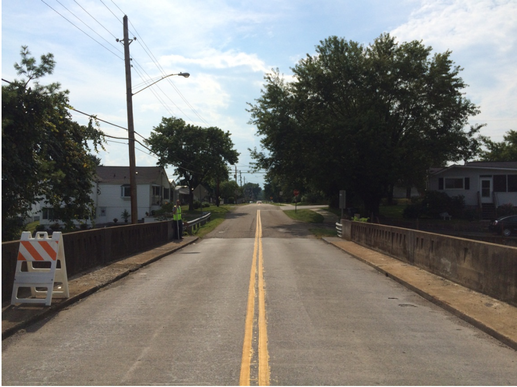
Center of Bridge Looking West on Local Route 03899
