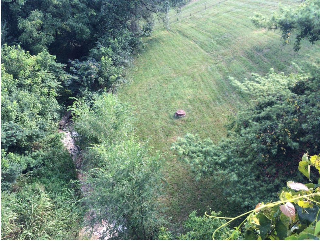
Man Hole to the Right of Downstream
