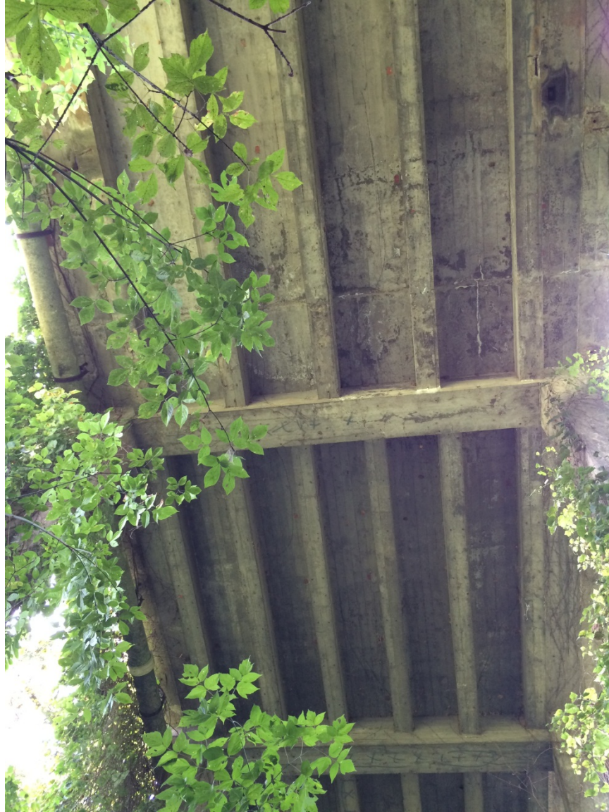
Underneath Bridge Deck
