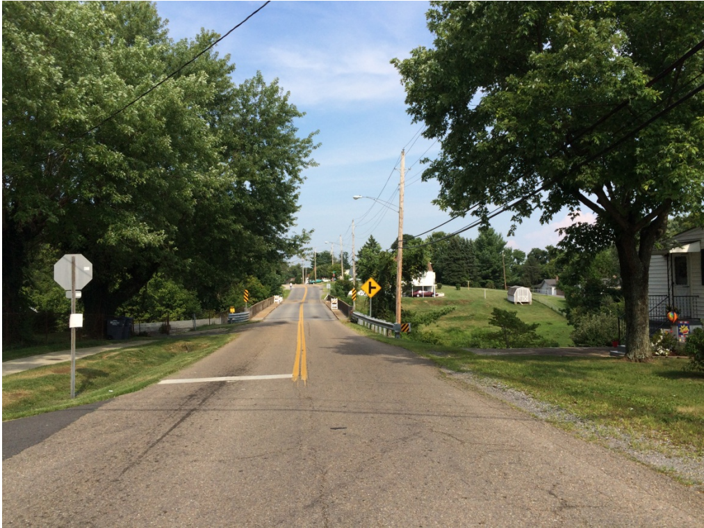
Eastbound Bridge Approach on Local Route 03899
